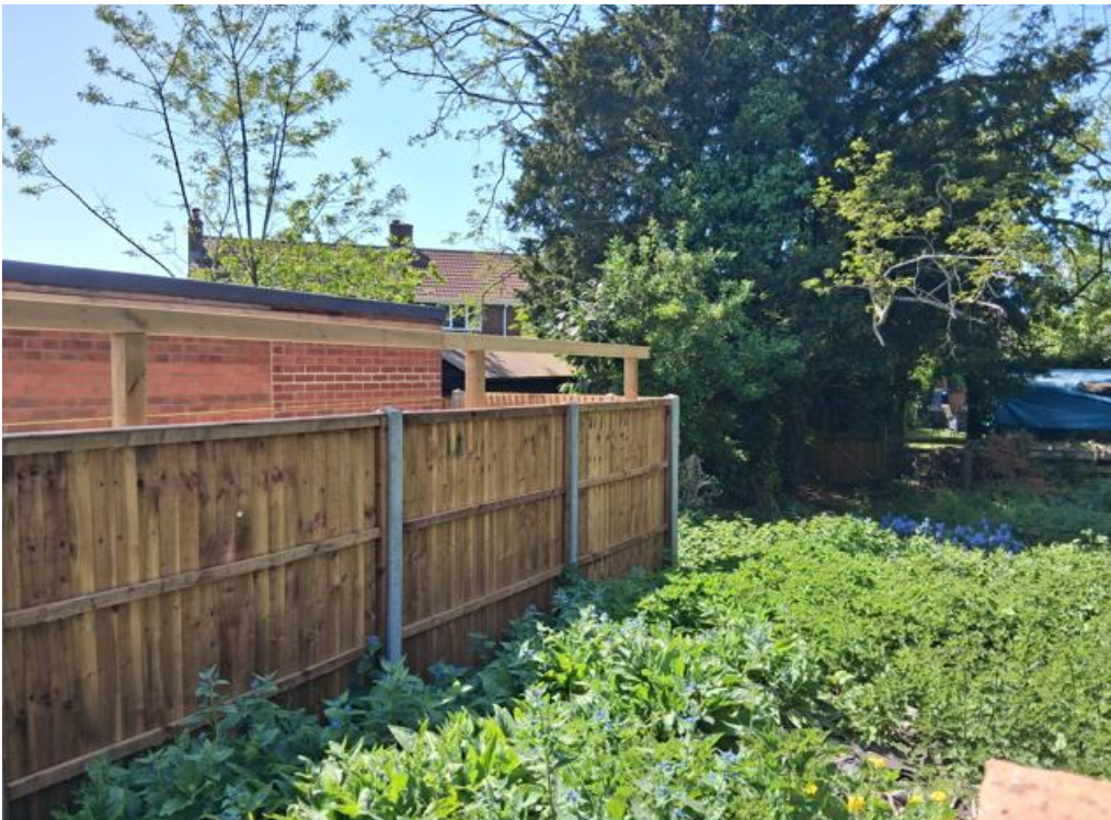
Photograph 6: View from Parker Court looking south to the site
