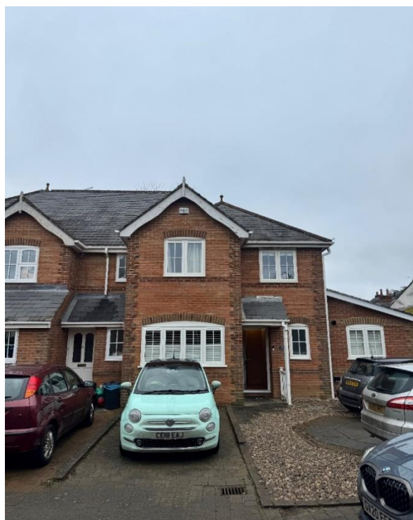
Street view of 7 Old Mill Court
