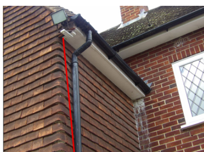
Figure 9. Gap in soffit on rear elevation. 3 Old Bath Road, Sonning. 20.01.26
