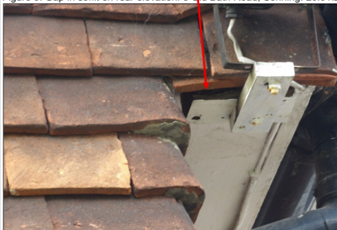
Figure 9. Gap in soffit on rear elevation. 3 Old Bath Road, Sonning. 20.01.26
