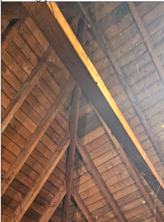
Photograph 7: Timber clad roof liner
