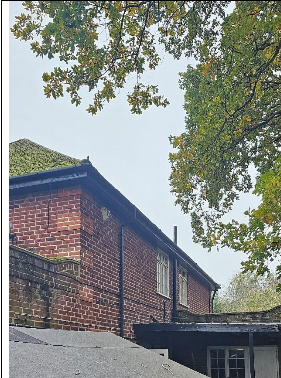
Photograph 5: Well fitted tight soffits without gaps.
