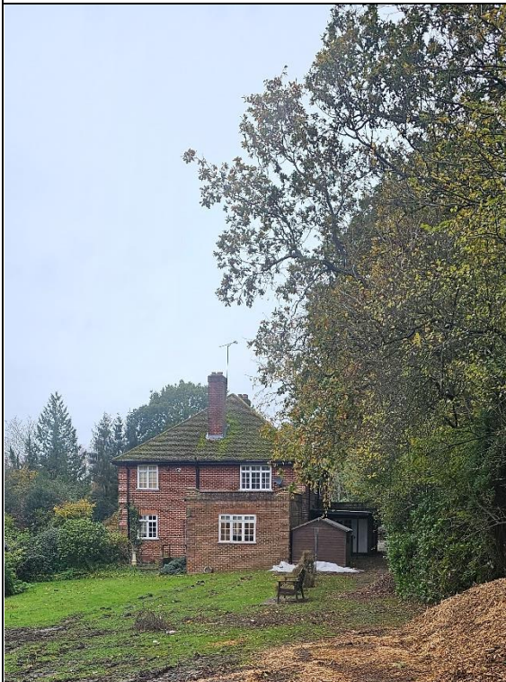
Photograph 3: Rear elevation of house.
