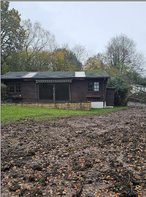
Photograph 1: Timber clad shed.
