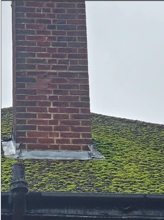
Photograph 9: Tight fitted lead flashing.
