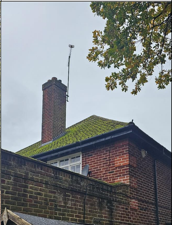
Photograph 4: Interlocking roof tiles in good condition no lifting or gaps.
