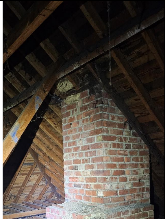
Photograph 6: Loft fully inspected.
