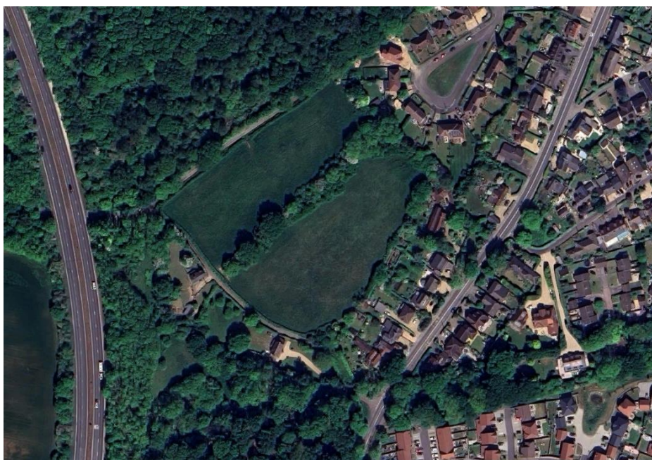
Image 1 – Land adjacent to Bull Lane and Sun Lane, Riseley
