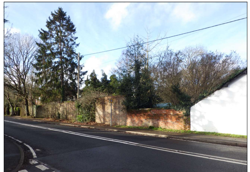
Plate 9: View looking west towards the application site with the boundary to Pound House (LB1) in the foreground
