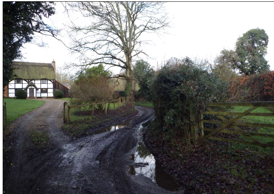
Plate 12: View looking northwest on approach towards Coldharbour Cottage (LB2) from Sun Lane, with the application site to the right
