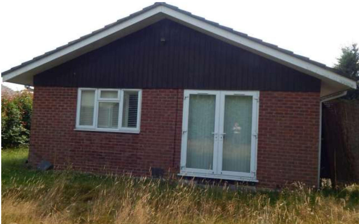
Image 2 – North facing elevation of the main dwelling
