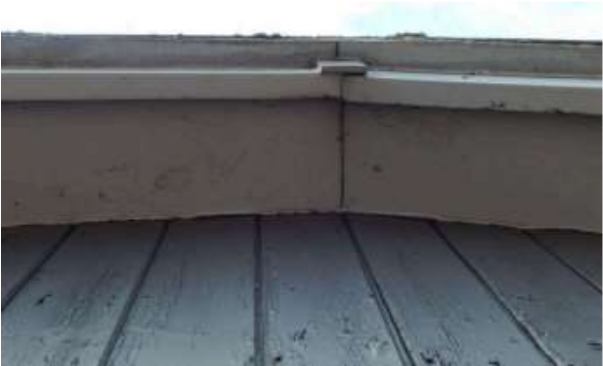
Image 7 – Close view of eaves coverings to the main dwelling
