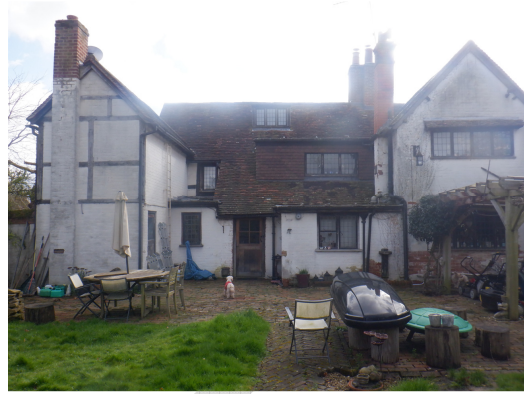
Photograph 2. Rear of property viewed from north.
