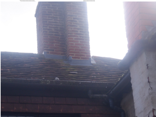
Photograph 10. Lead flashing sealed to brick chimney and clay tiles (rear elevation)
