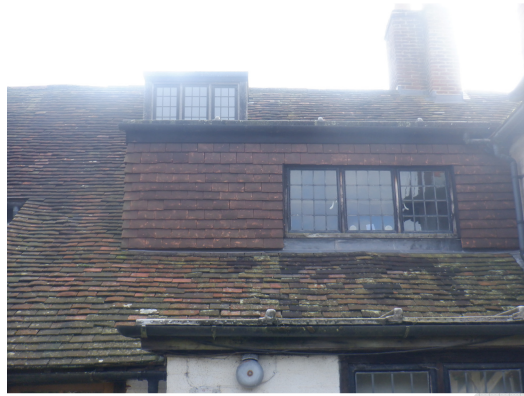
Photograph 12. Dormer clad with hanging tiles (rear elevation).
