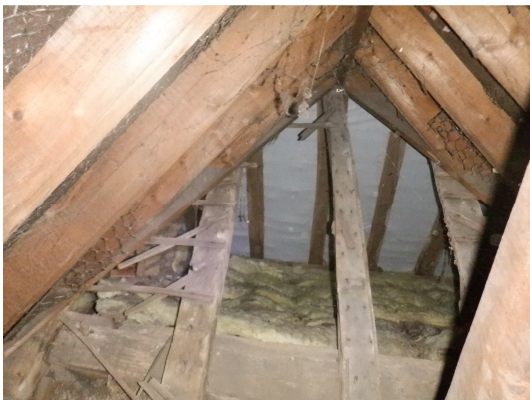
Photograph 20. Original roof trusses visible and allowing access to the western half of Roof void 2.
