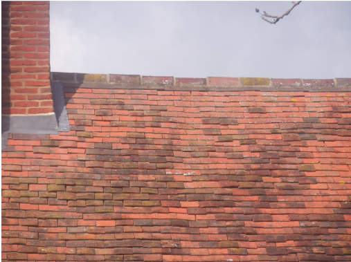
Photograph 7. Ridge mortar fully intact (front elevation)
