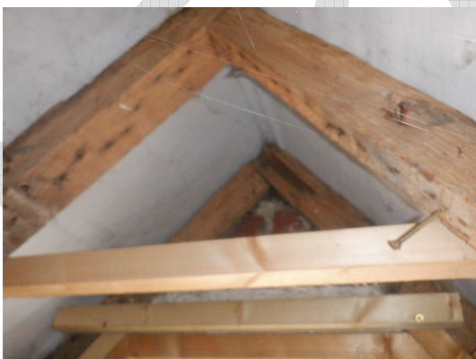
Photograph 22. Breathable roofing membrane fully intact throughout (Roof void 2).
