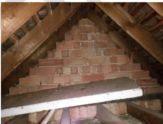
Photograph 18. Fibreglass insulation at the edges of the eastern brick gable (Roof void 1).
