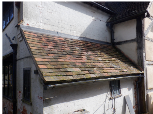
Photograph 11. Lead flashing sealed along wall (west elevation).
