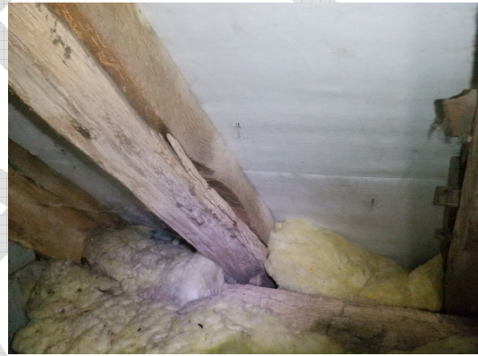
Photograph 25. Eaves filled with fibreglass insulation.
