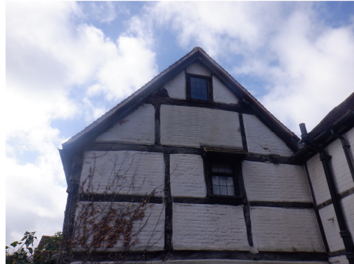
Photograph 8. Recently mortared verge (east elevation).
