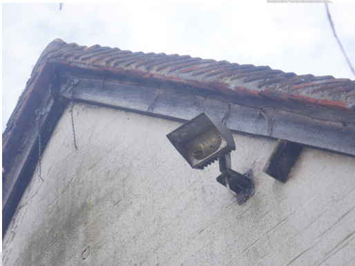
Photograph 13. Timber fascia sealed to the painted brickwork gable (rear elevation).
