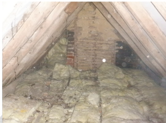
Photograph 21. Roof void 2 looking towards the central chimney.
