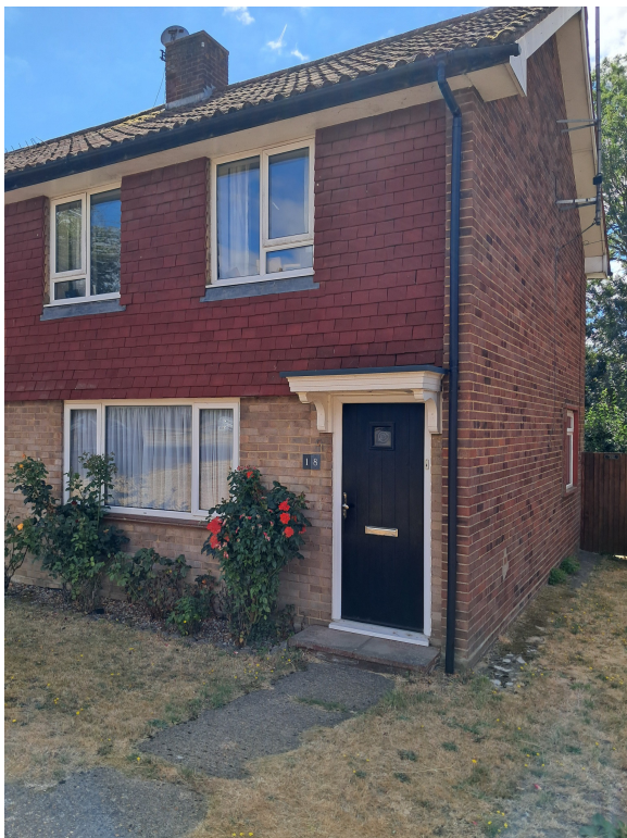
Front Elevation – general view
