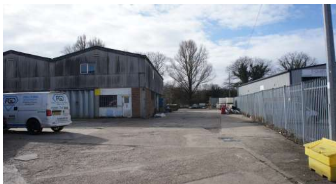
View from within the Site looking south
