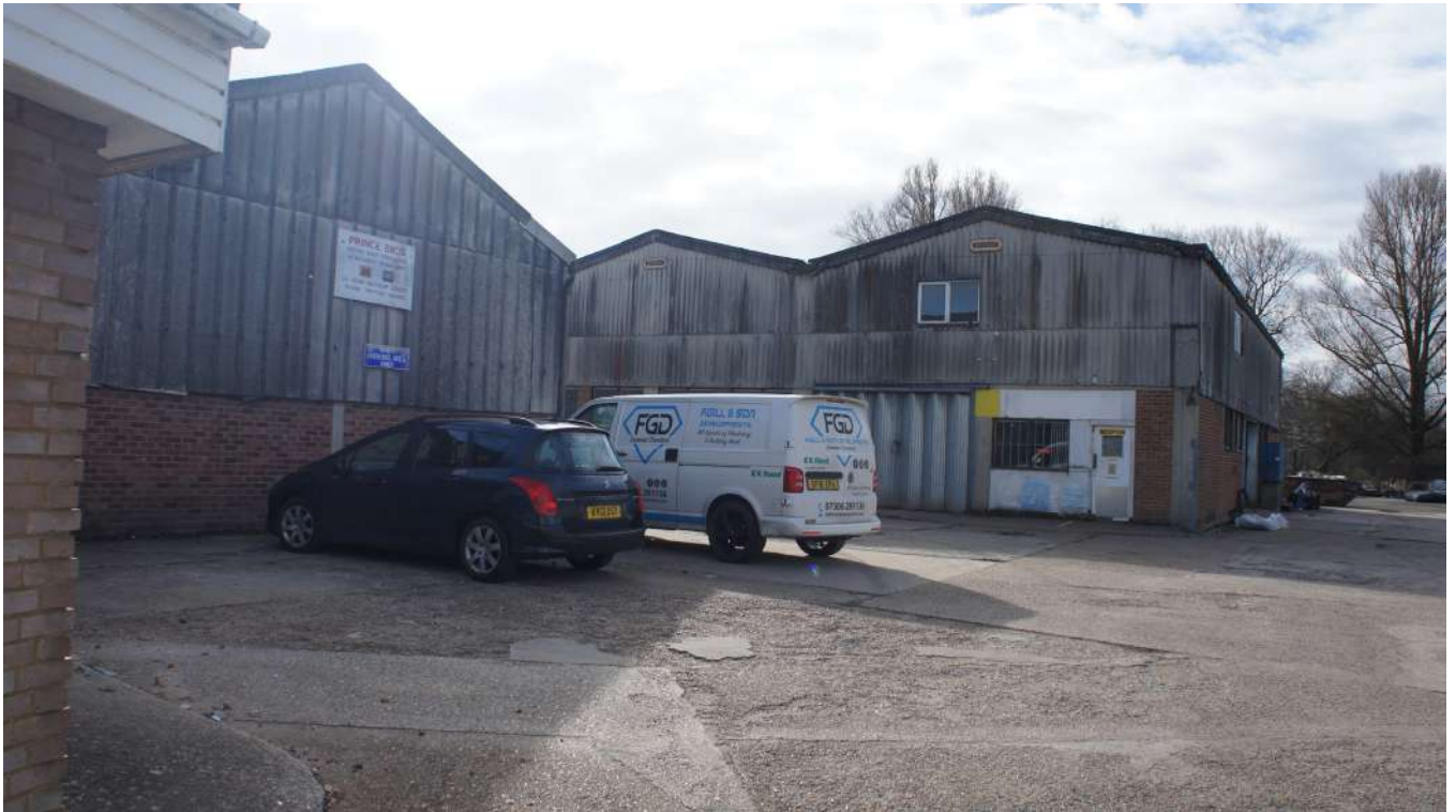
2 View into site from site entrance
