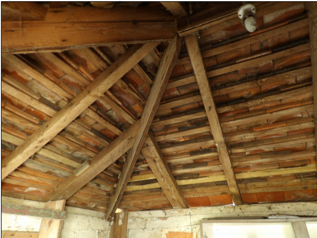
Figure 16. Interior of outbuilding. 5 Walden Avenue, Arborfield. 25.02.25
