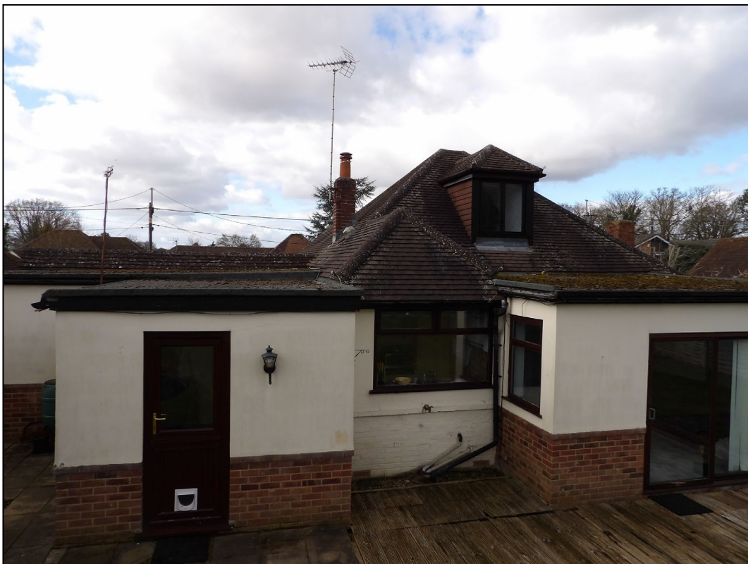
Figure 7. Rear, flat roof extensions. 5 Walden Avenue, Arborfield. 25.02.25
