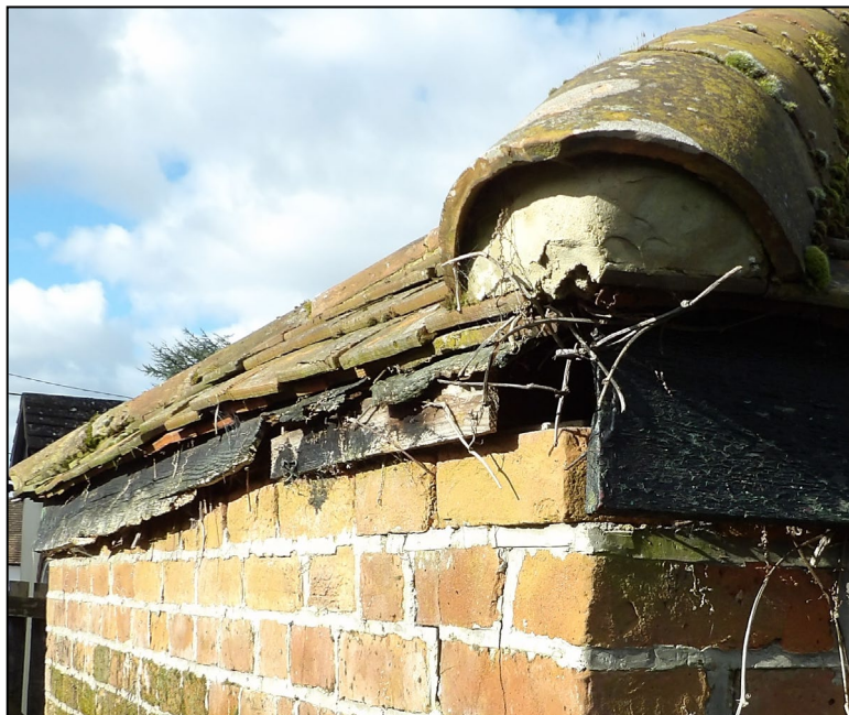
Figure 12. Rear view of moved tiles and rotten fascia on outbuilding. 5 Walden Avenue, Arborfield. 25.02.25
