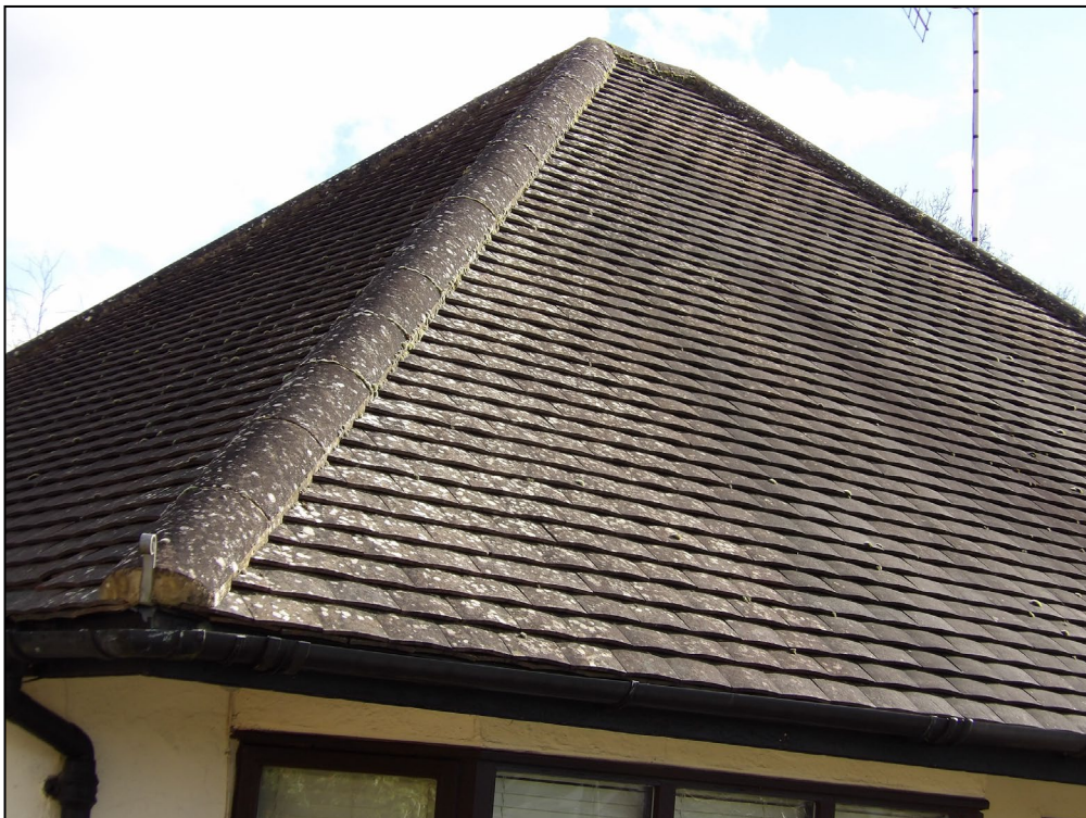
Figure 5. Example sealed ridge and hip tiles. 5 Walden Avenue, Arborfield. 25.02.25
