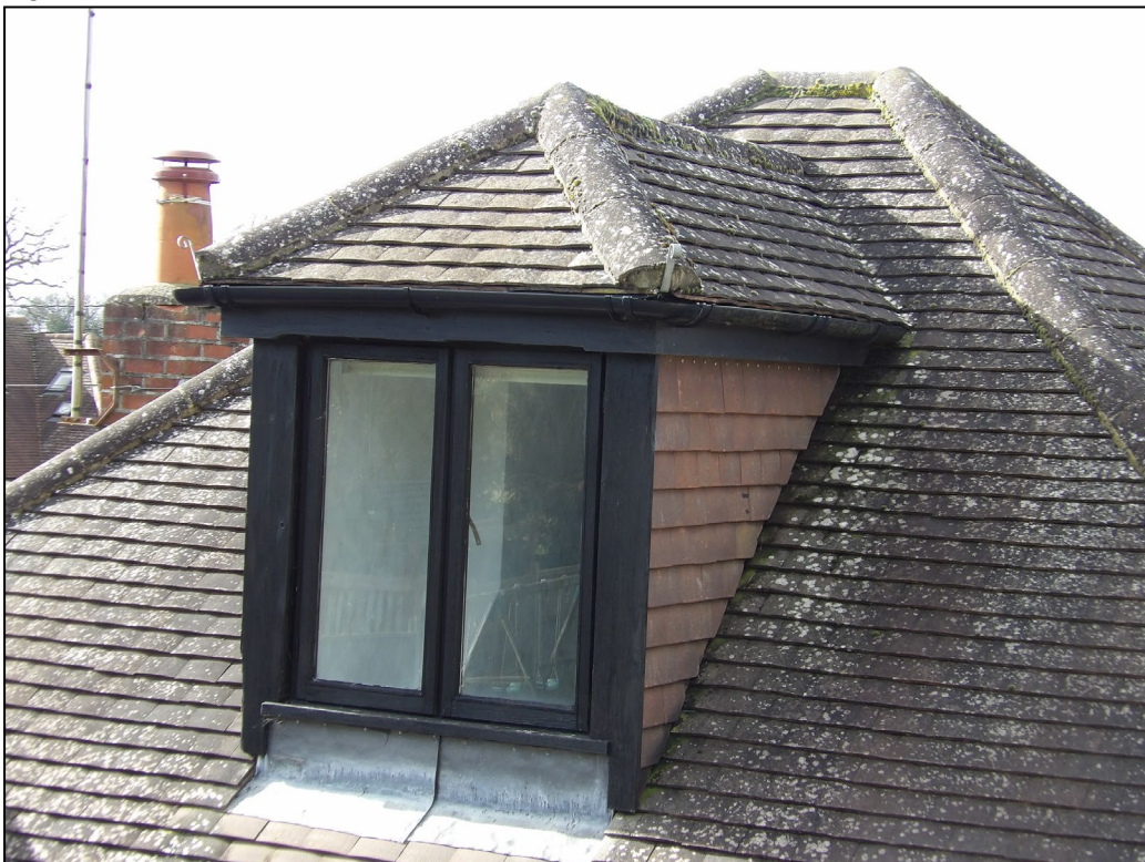
Figure 9. Dormer window on rear elevation. 5 Walden Avenue, Arborfield. 25.02.25
