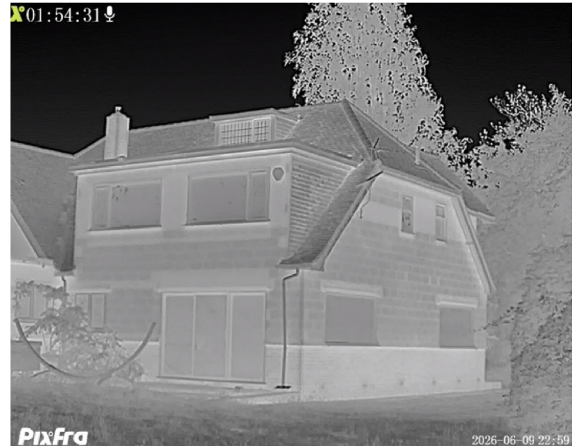
Pixfra ARC A613 at Surveyor Location 2.
