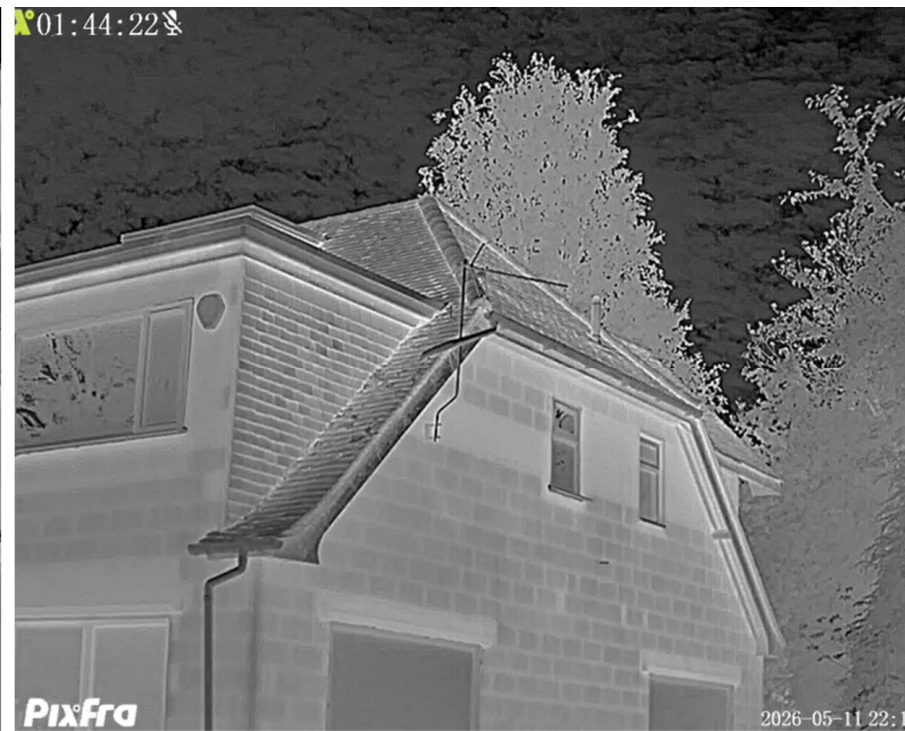
Pixfra ARC A613 at Surveyor Location 2.
