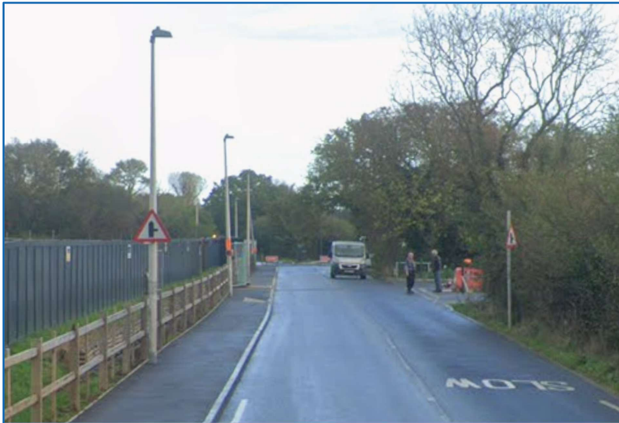
Figure 3 - Baseline Lighting along Cutbush Lane East (Google Maps, November 2022)
