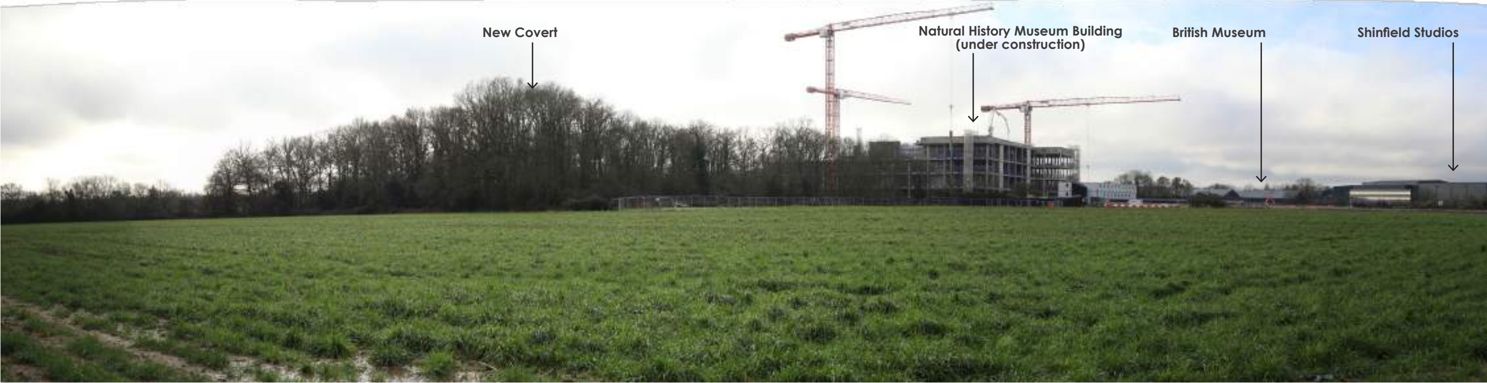
View E: From north-east of New Covert, looking towards the western end of the proposed track. The track will run close to this northern boundary of New Covert, with the NHM building iunder construction a dominant feature in the view.
