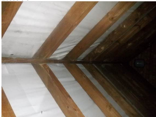
Photograph 19. The roof space was lightly cobwebbed.
