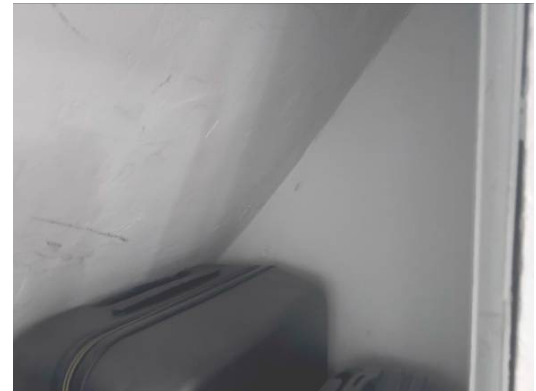
Photograph 14. Eave space plastered out and carpeted.
