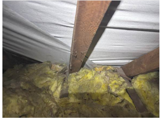
Photograph 16. Thick fiberglass insulation which filled the eaves.
