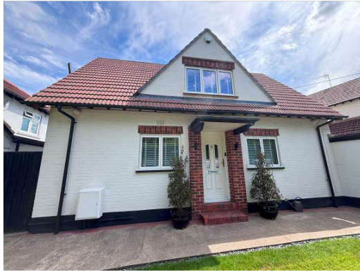
Photograph 1. Front of property viewed from the north.
