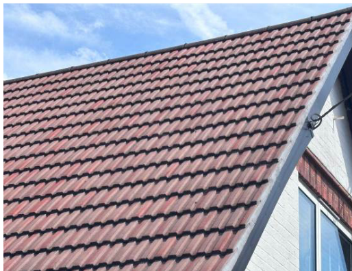
Photograph 4. Tightly fitted roof tiles at the front (northern) side of the property.
