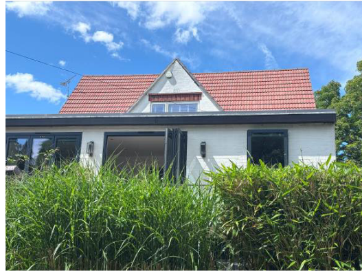
Photograph 2. Rear of property viewed from the south.
