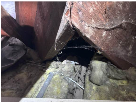
Photograph 17. Rear gable end visible but not accessible.
