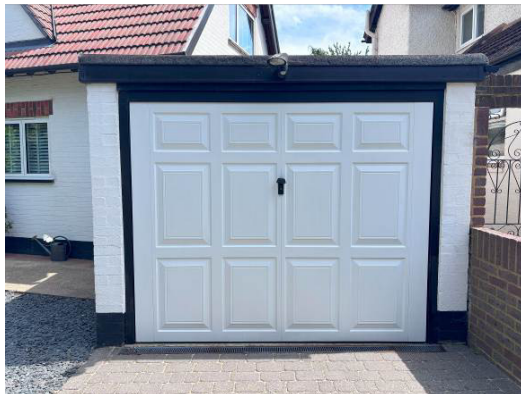
Photograph 3. Garage attached to the western side of the house.
