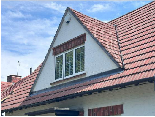
Photograph 6. Verges mortar intact at the verges to the front of the property
