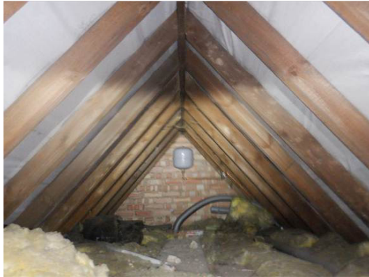
Photograph 15. Roof space of gable end construction and lined with breathable roofing membrane.
