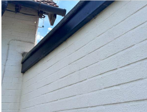
Photograph 11. Garage roof tightly fitted.
