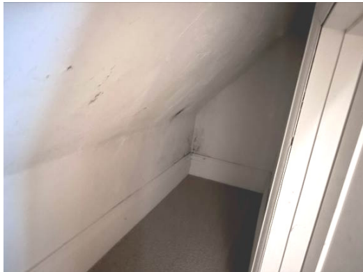
Photograph 13. Eave space plastered out and carpeted.
