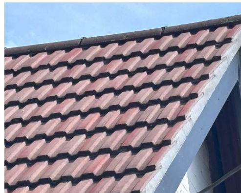
Photograph 5. Tightly fitted dry ridge fix system
