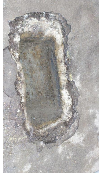
Photograph 8 - Looking down at TP02.
