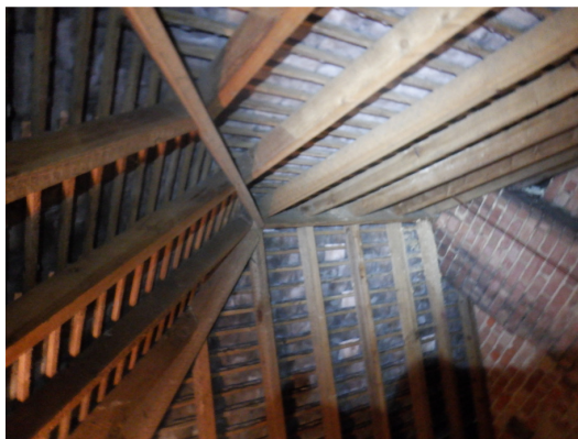
Photograph 13. Unlined roof in roof void.
