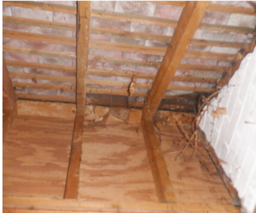
Photograph 20. Unlined roof and wall clad with timber towards the front of the garage.
