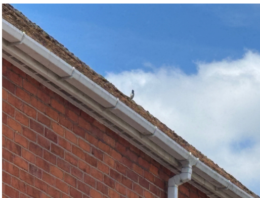
Photograph 6. Soffit boxes tight to the brickwork
