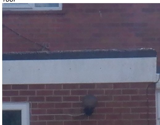
Photograph 11. uPVC barge boards tight to rear (west facing) brick work and roofing of the single storey extension.
