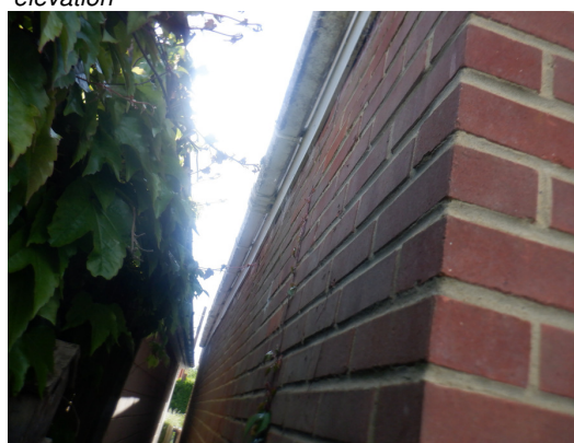
Photograph 10. Intact and tight barge boards around garage (northern elevation).
