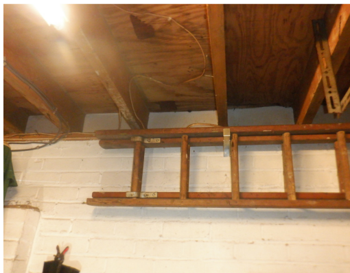
Photograph 18. Timbers tight to the brick walls in the flat roofed section of the garage.
