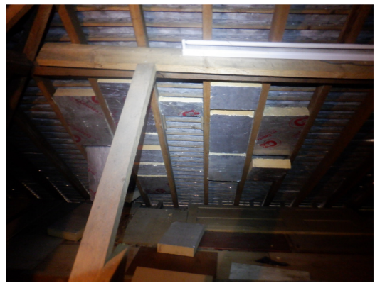
Photograph 14. Small section of roof with foil boards.
