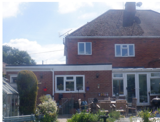
Photograph 2. Rear of the house viewed from the west.
