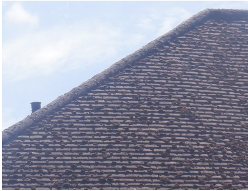
Photograph 3. Tight/flat plain roof tiles and intact hip tiles (rear elevation)
