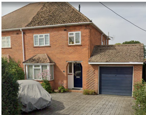
Photograph 1. Front of the house viewed from the east.
