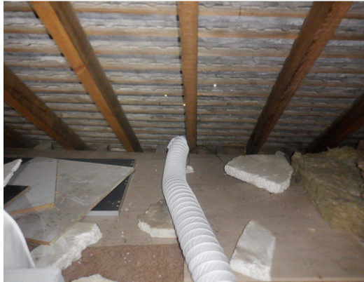
Photograph 15. Boarded and carpeted floor with thick fibreglass underneath boarding.
