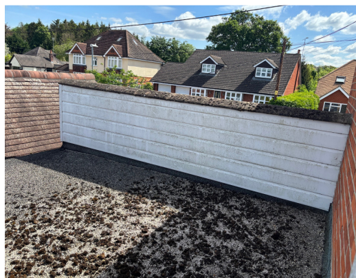
Photograph 9. uPVC backing of garage sloped roof
