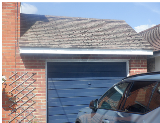
Photograph 8. Garage sloped roof (front eastern elevation)
