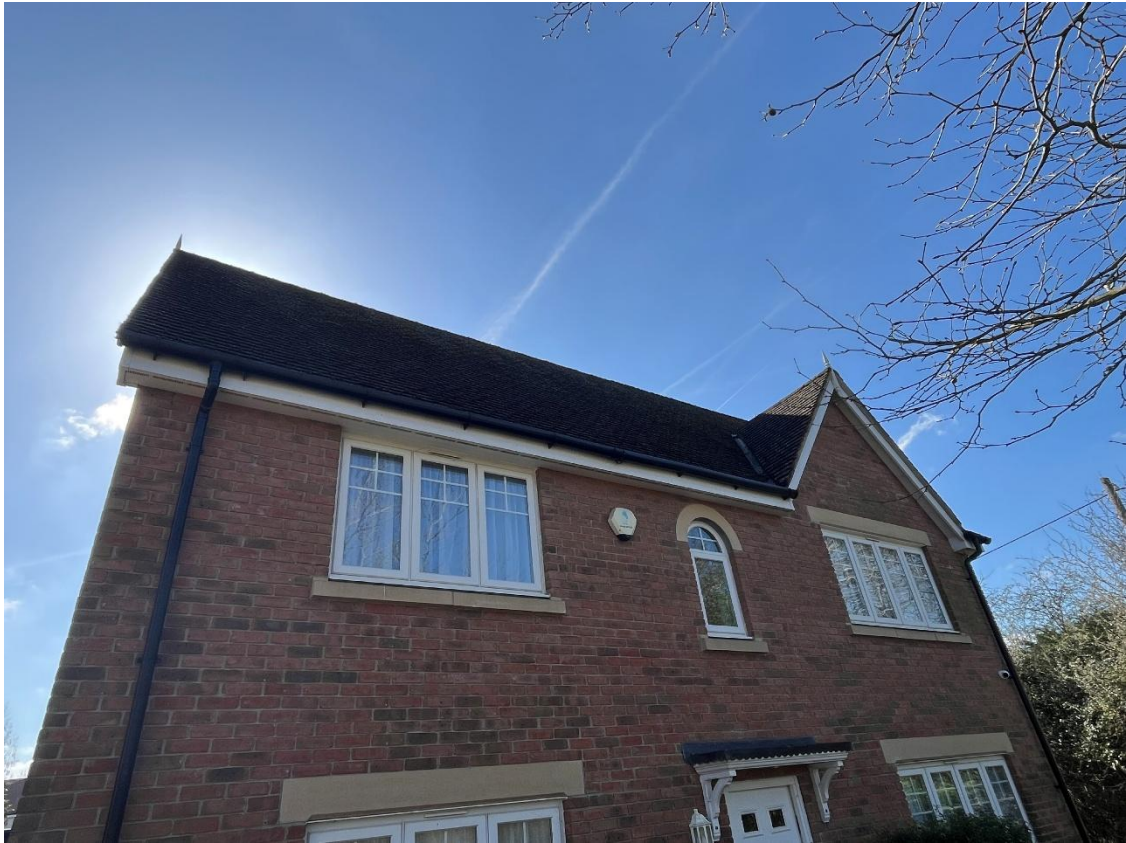
Figure 3. Northern elevation looking southwest
