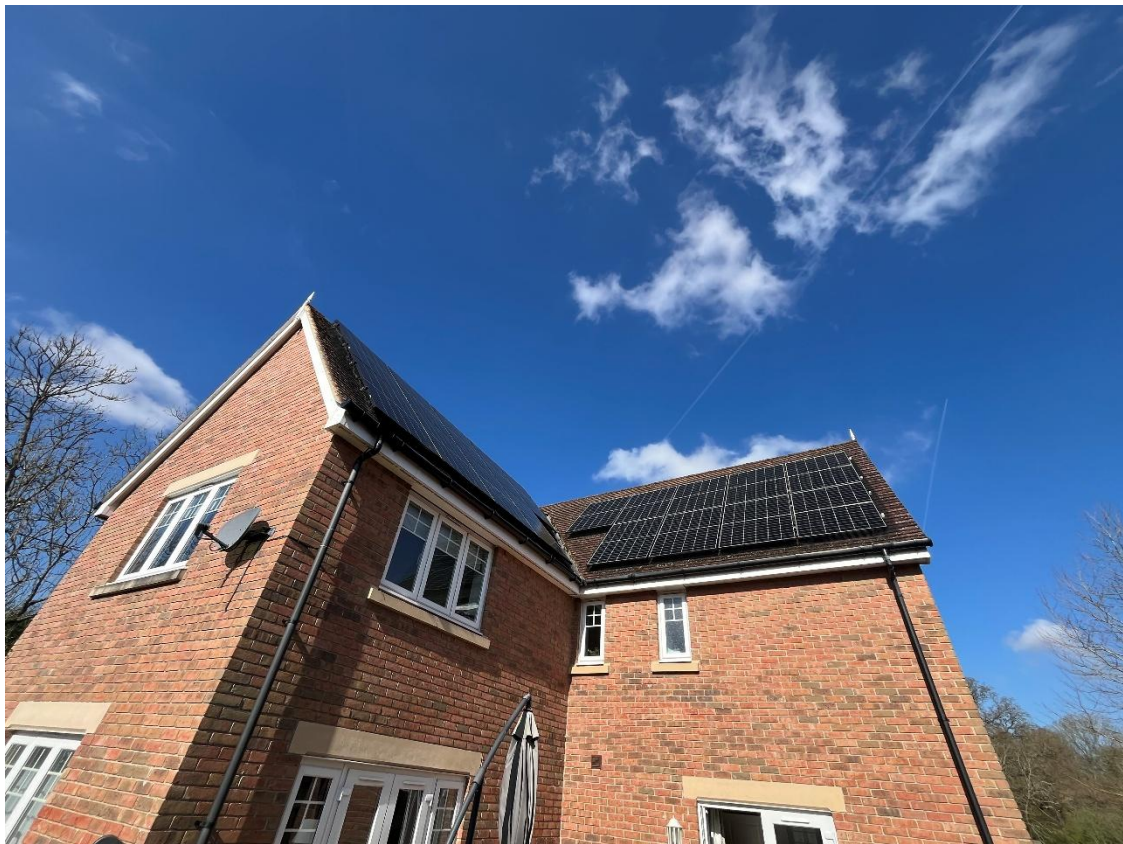
Figure 4. Southern and eastern elevations looking north
