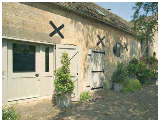
Figure 8.14: Retention of original features such as the stable joinery in this example is important to retain the character of the building
