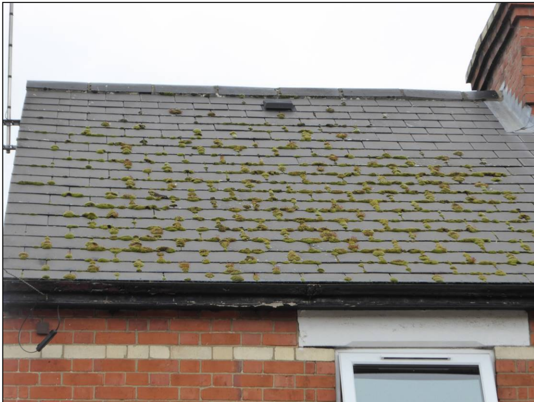
Figure 4. Example of roof tiles. 1 Diamond Villas, The Street, Hurst. 05.03.21
