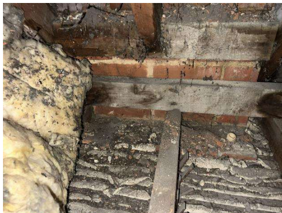
Photograph 06 – Chimney extended down into boxing location from roof void
