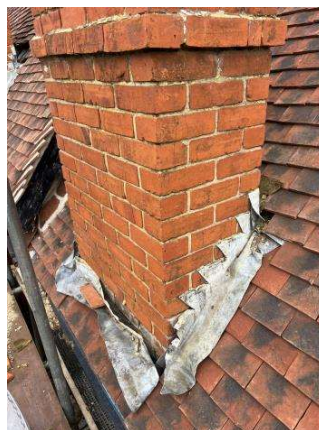
Photograph 01 – Existing lead flashing around base of the chimney
