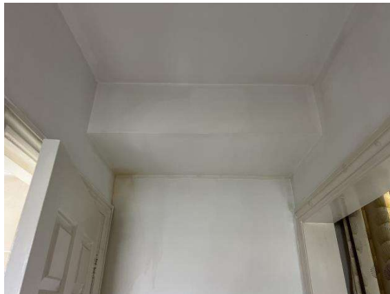
Photographs 04 & 05 – Structural support for chimney likely concealed with ceiling boxing in both the first floor bathroom and landing
