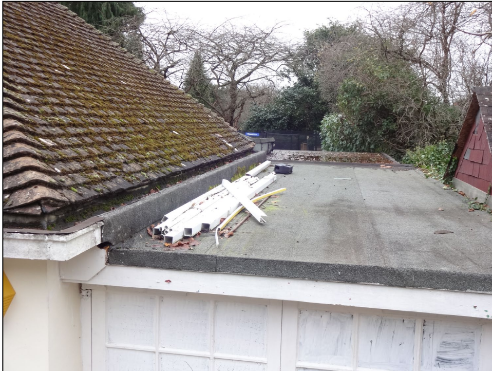
Figure 11. Bitumen covering garage roof. Fernlea, 1 Garde Road, Sonning. 16.12.21
