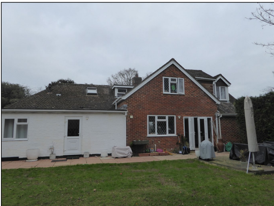
Figure 6. View of rear of property showing flat roof section. Fernlea, 1 Garde Road, Sonning. 16.12.21
