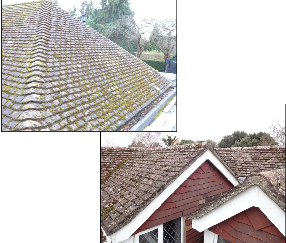
Figure 5. Example of ridge/hip tiles and sealed verges. Fernlea, 1 Garde Road, Sonning. 16.12.21
