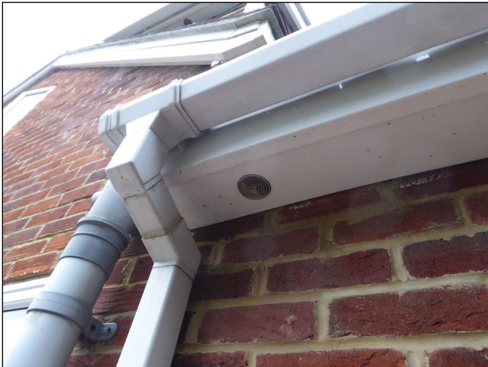
Figure 8. Example soffits/fascias. Fernlea, 1 Garde Road, Sonning. 16.12.21
