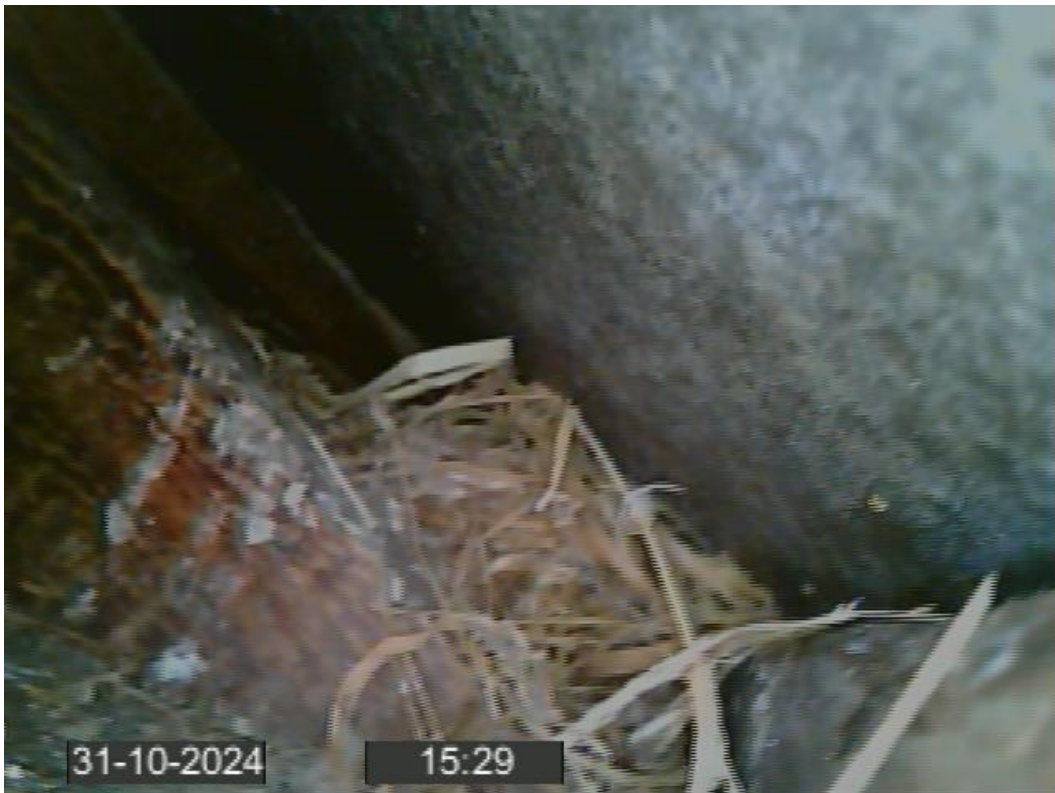
Photos 13 and 14 – Photos from endoscope inspection of Features D and E
