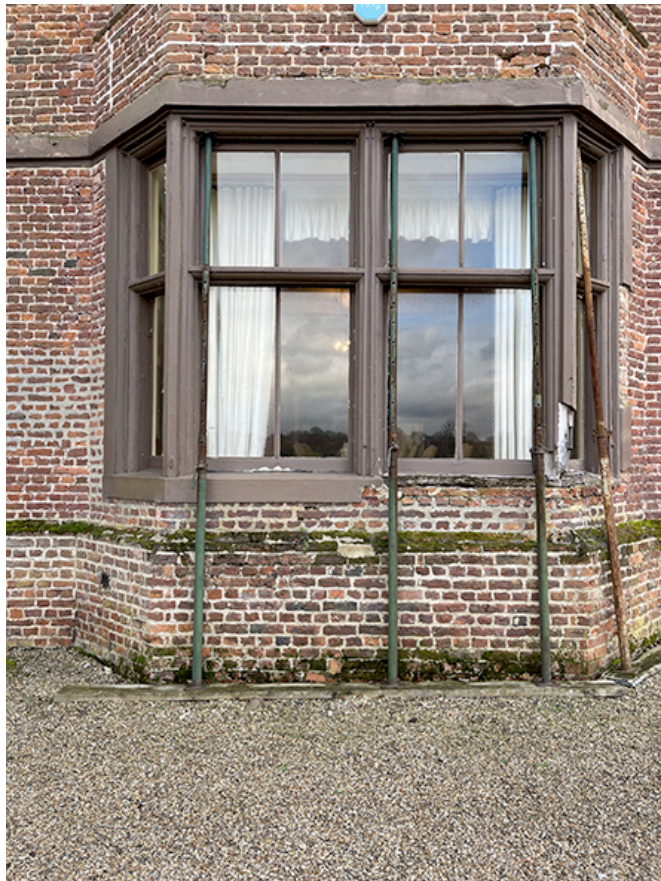
Ground floor north bay
