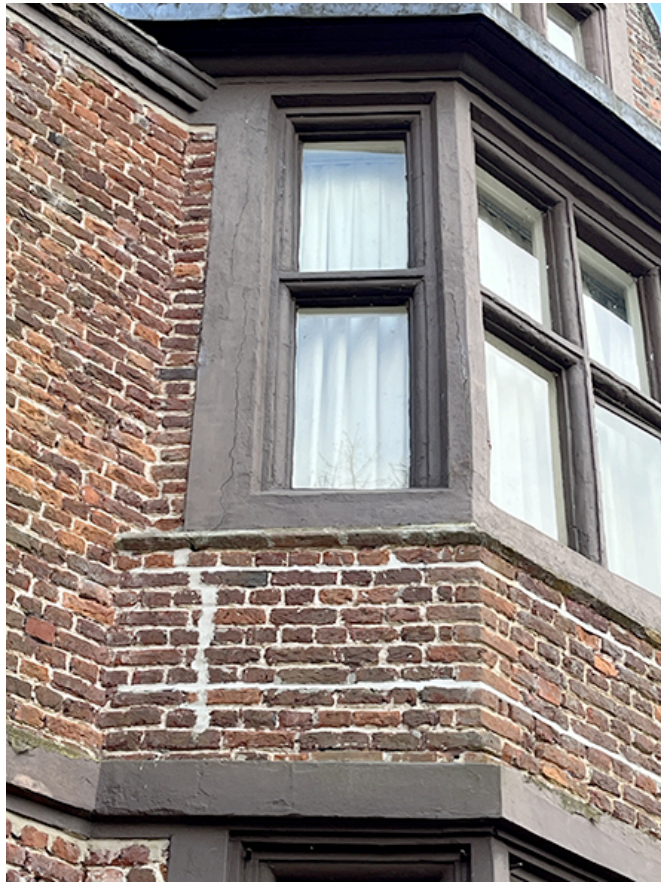
1st floor north bay
