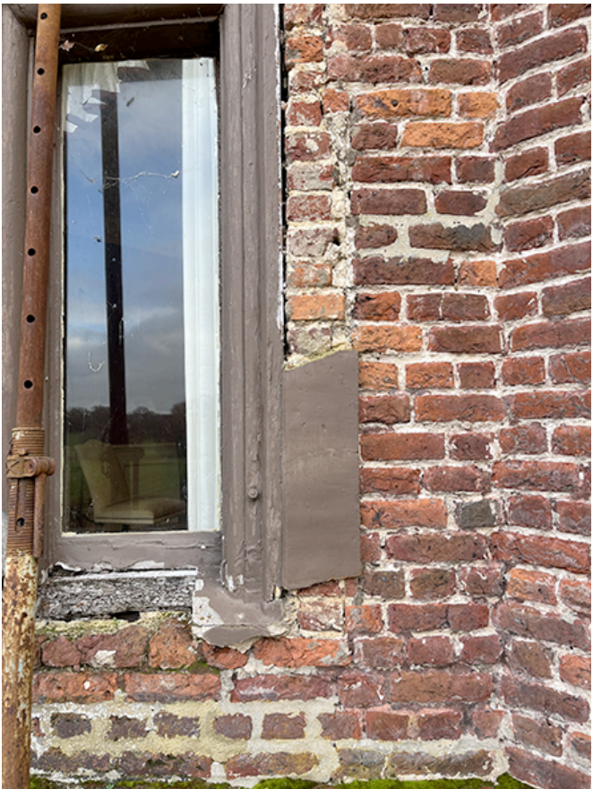
Ground floor north bay
