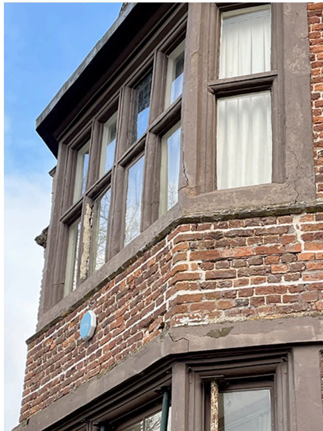
1st floor north bay
