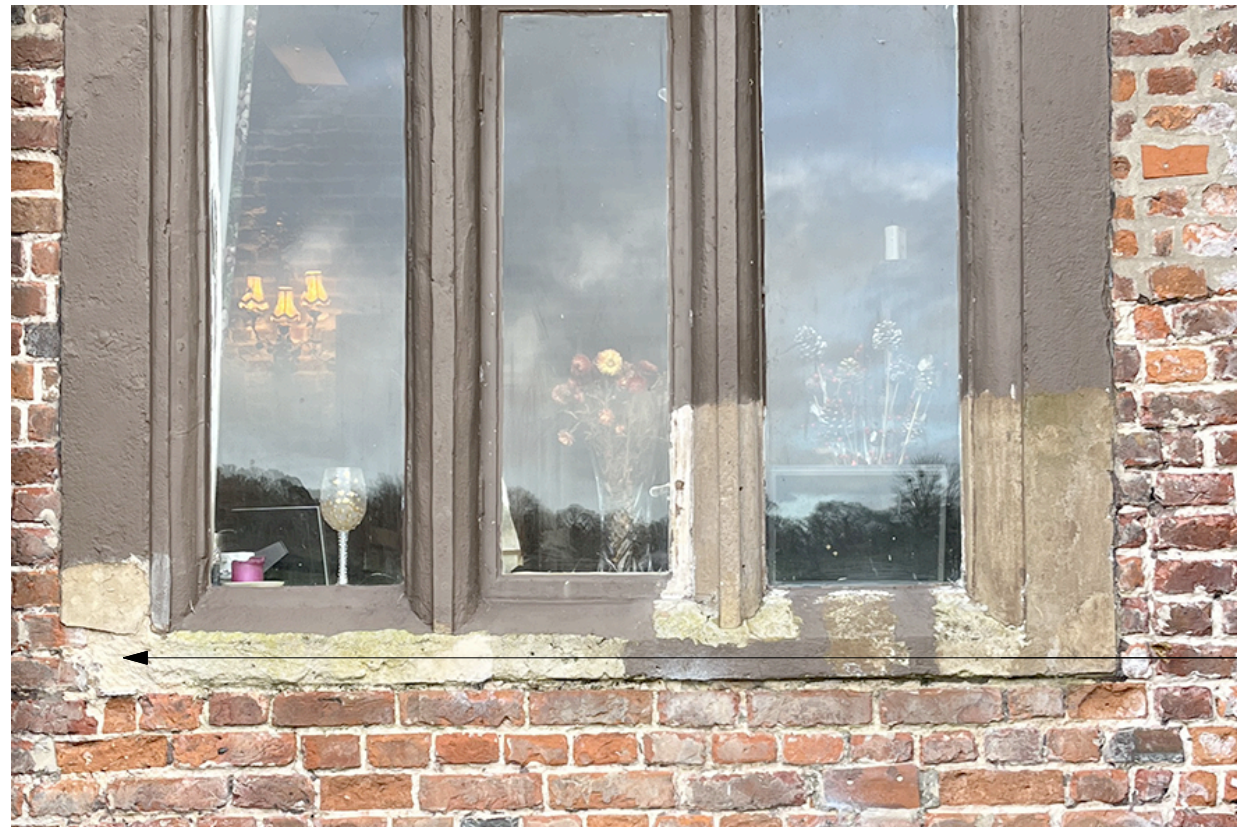
Ground and 1st floor south bay Victorian 1 over 1 sash windows
