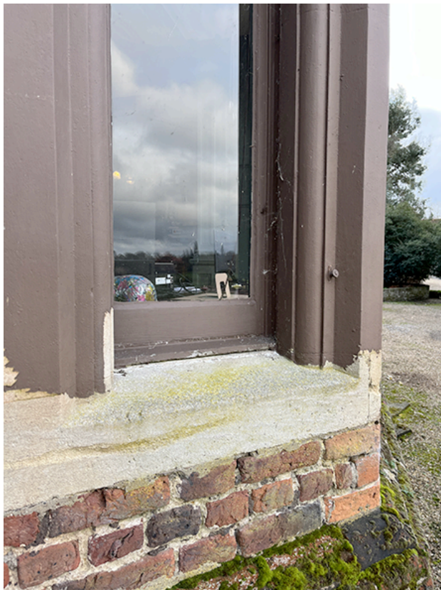
Ground floor south bay Victorian 1 over 1 sash windows
