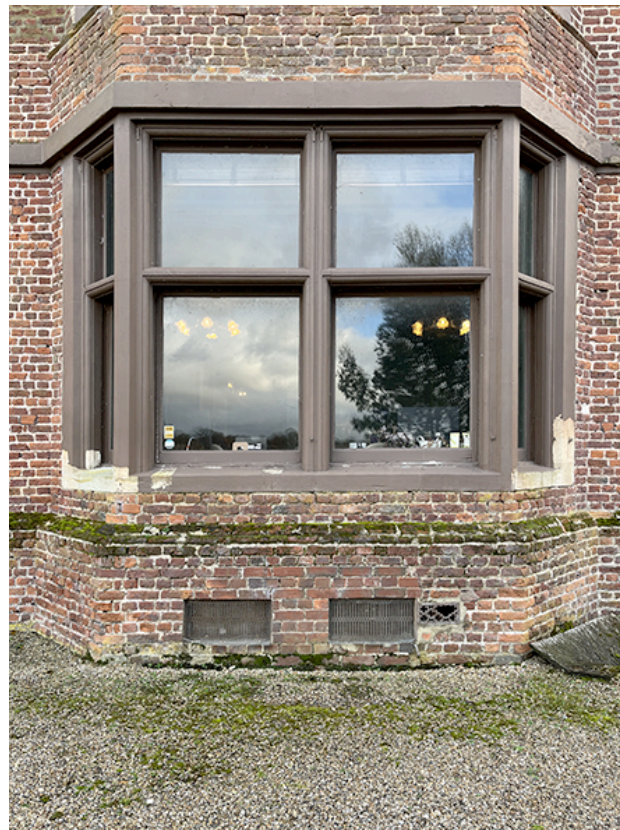
Ground and 1st floor south bay Victorian 1 over 1 sash windows
