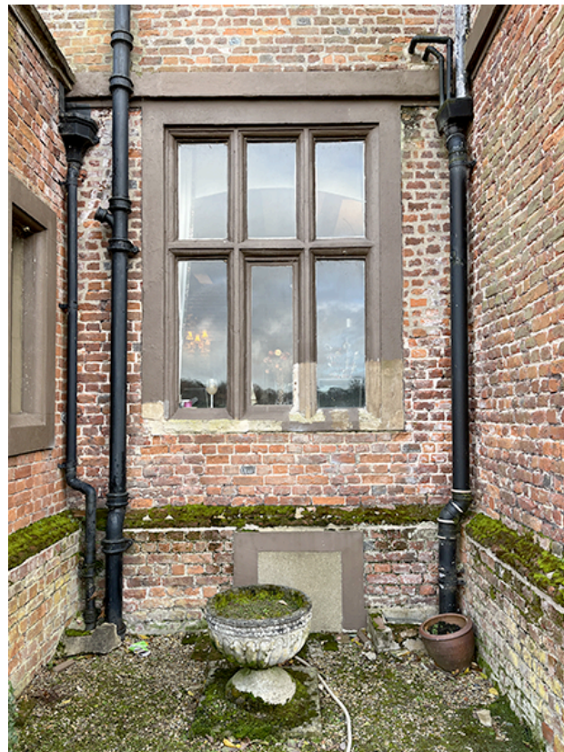
Ground floor window south of entrance Showing stone window surround
