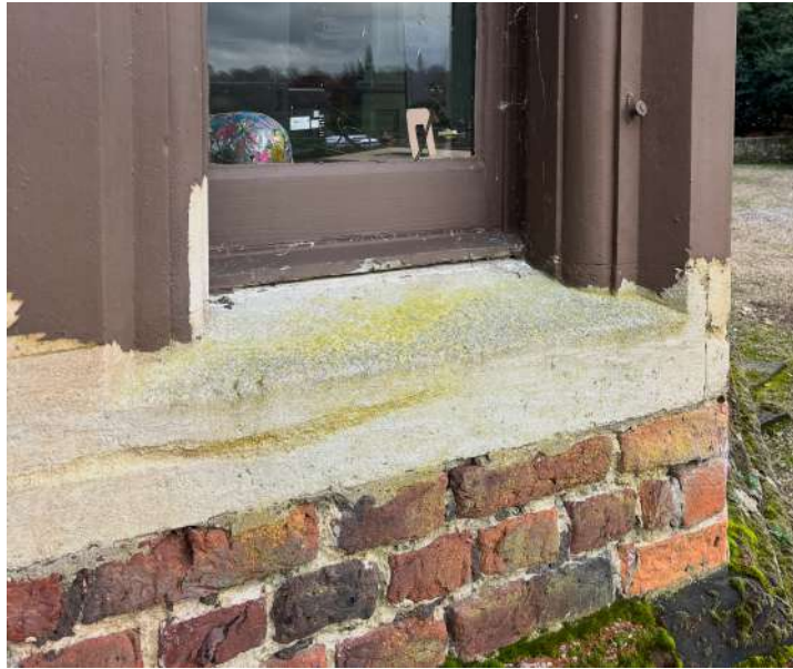
Right hand bay, ground floor, showing unpainted sandstone, painted sandstone mullions, and painted Victorian/Edwardian sash window
