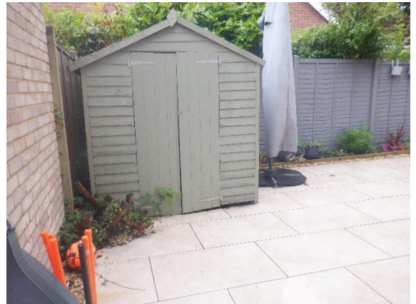
4. Timber shed in southern corner of the garden (u1b5)
