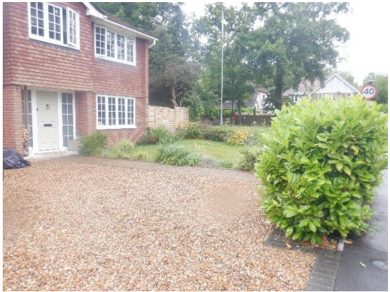
3. Main house viewed from the east (u1b5)
