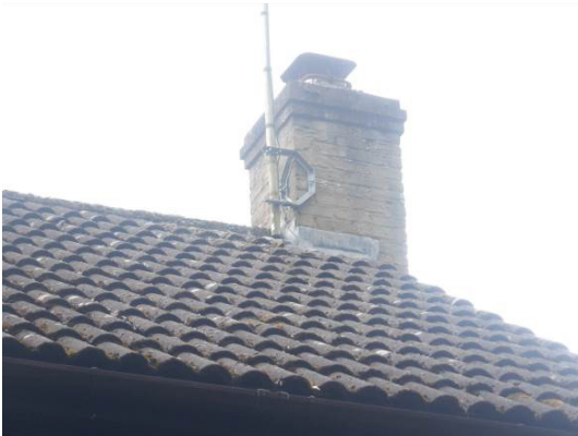
Photograph 3. Intact interlocking tiles.
