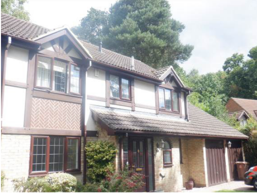
Photograph 1. Front of property viewed from southwest.
