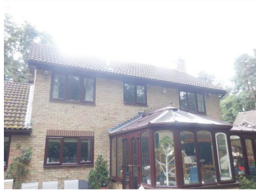
Photograph 2. Rear of property viewed from north.
