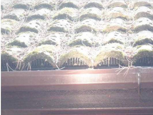
Photograph 10. Intact interlocking tiles and mesh at the eaves (southern elevation).
