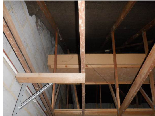
Photograph 24. Internal wall of block work construction (western elevation).
