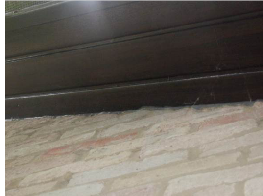
Photograph 11. Sealant filling part of the eaves (eastern elevation).
