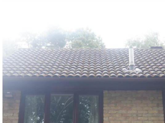
Photograph 4. Ridge mortar intact.
