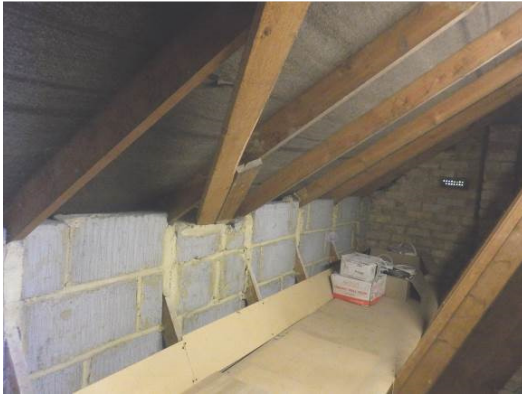
Photograph 23. Garage lined with bitumen roofing felt with block work at the eaves.
