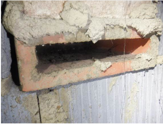
Photograph 18. Heavily cobwebbed ventilation brick in the gable end.
