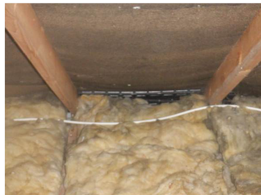
Photograph 14. Plastic ventilation at the eaves.
