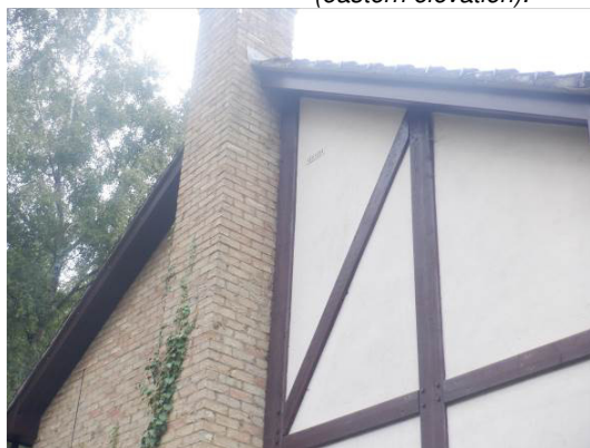
Photograph 9. Verge mortar intact (eastern elevation).
