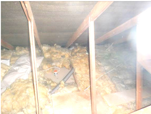
Photograph 16. Eaves filled with fibreglass (roof void).
