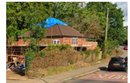
PRE-EXISTING FENCE WATERLOO COTTAGE (DURING CONSTRUCTION)
