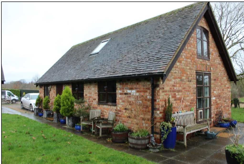
Photograph 1 – Side elevation as viewed from the garden
