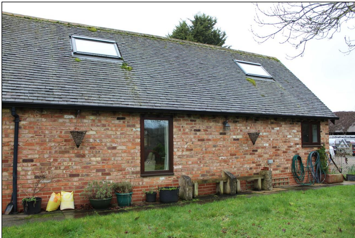
Photograph 2 – Side elevation showing area of proposed new extension
