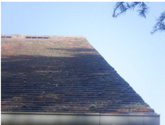
Photograph 16. Roof tiles lifted towards the verge on the pitched roof attached to the south western end of the flat roof building (south eastern elevation).
