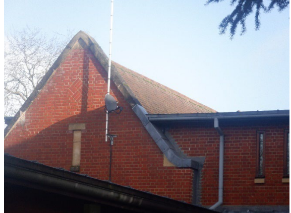
Photograph 14. Concrete tile ends and lead flashing on the gable end and flat metal roof all tight.
