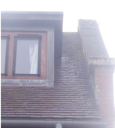
Photograph 13. Tight roof tiles and concrete around the gable end wall at the northern eastern end of the building (north western elevation).
