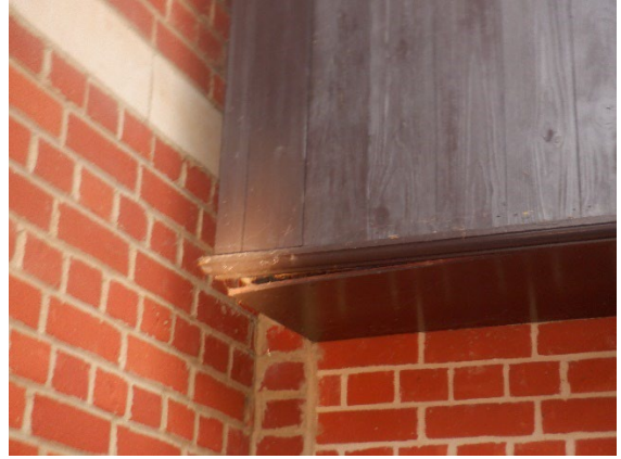
Photograph 11. Gap at base of timber soffits (north western elevation).
