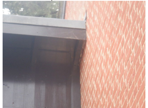
Photograph 8. Gap at edge of the roof between the roof and adjacent wall (north western elevation).
