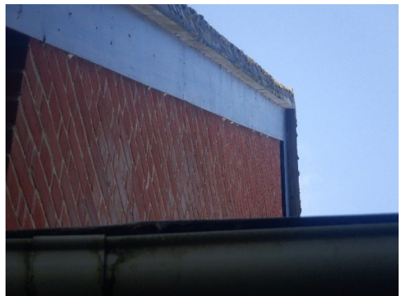
Photograph 17. Verge mortared and timber fascias tight to the wall attached to the south western end of the flat roof building.
