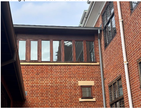
Photograph 15. Flat roof and adjoining roof of the main house tightly fitted with painted soffits.
