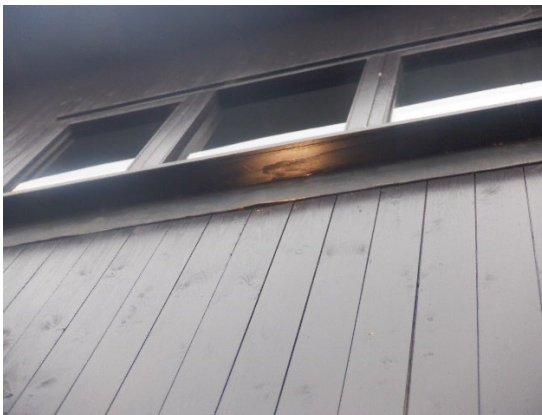
Photograph 12. Small gap behind lead flashing beneath a window (north western elevation).
