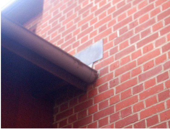
Photograph 10. Lead flashing tight to the wall at the eastern end of the building (south eastern elevation).
