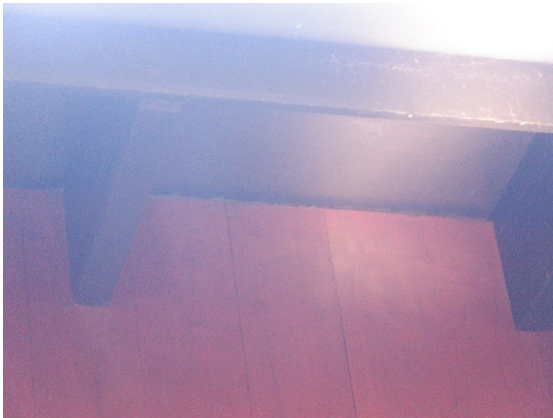
Photograph 7. Gaps beneath the timber soffits (south eastern elevation).
