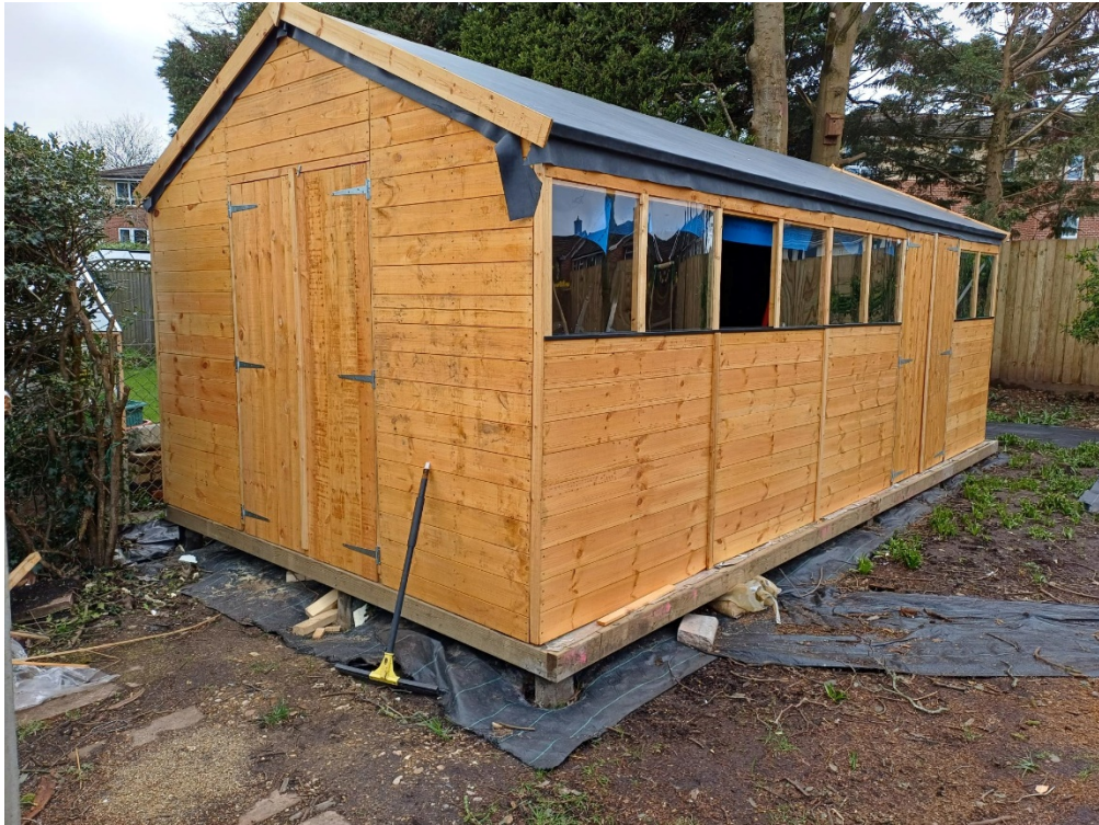
Shed Outbuilding (raised or on screws?)
