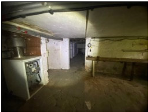
Figure 19 – Basement under the main house.
