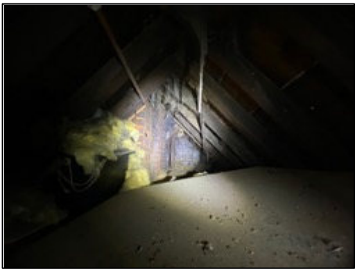
Figure 21 – Roof void 2 inside northern pitched roof.
