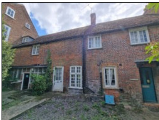
Figure 29 – Northern elevation of Rose Cottage.
