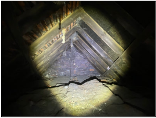
Figure 22 – Roof void 3 inside south-eastern roof pitch.
