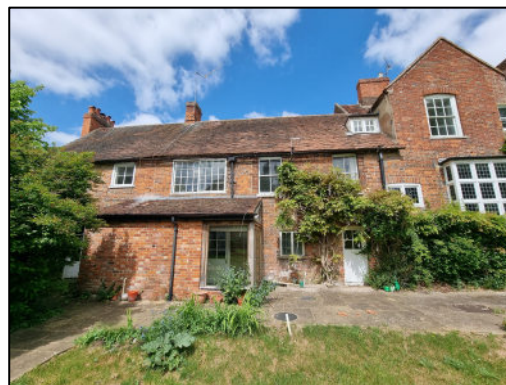
Figure 30 – Northern elevation of Rose Cottage.
