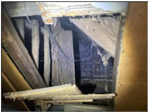
Figure 23 – Roof void 4 inside south-western roof pitch.
