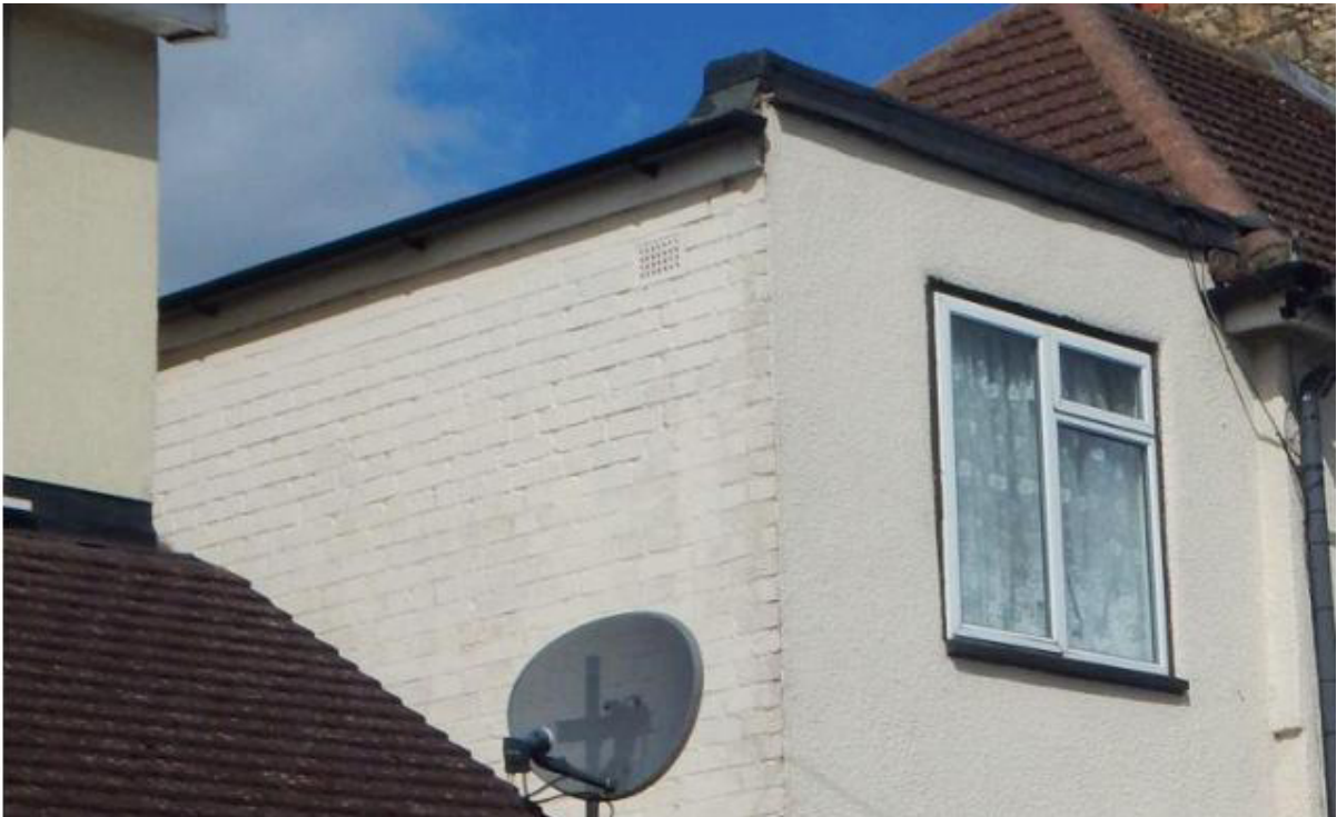
Image 3 – South facing elevation of the property
