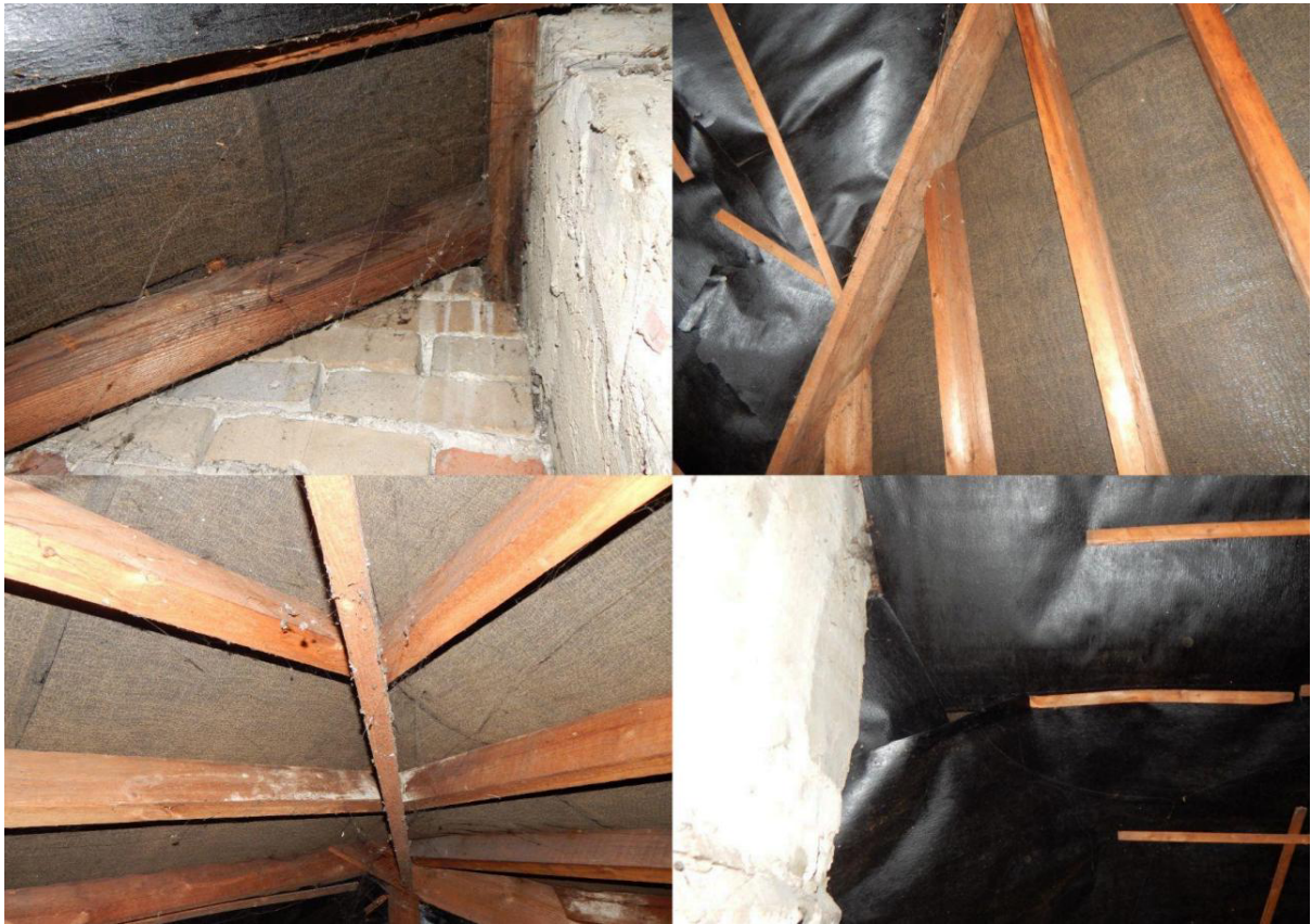
Image 9 – Internal view from within the main roof void spaces of the property
