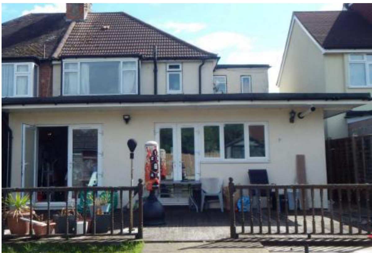
Image 2 – West facing elevation of the property
