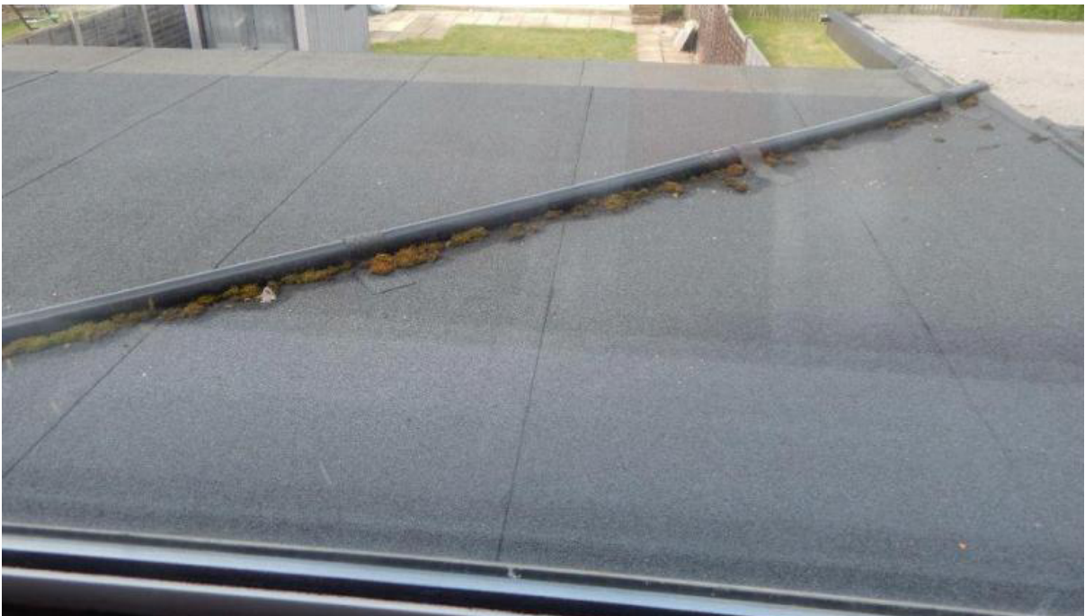
Image 4 – Views across the flat roof section of the property
