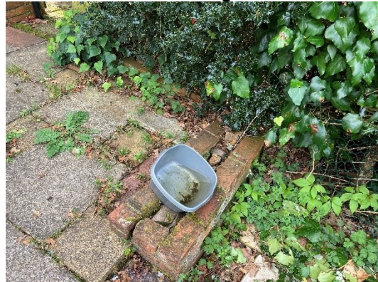
6. Loose bricks around the raised patio to the rear of the house.
