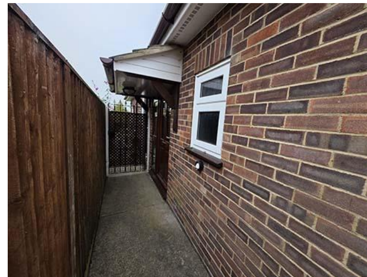
Existing entrance to north elevation
