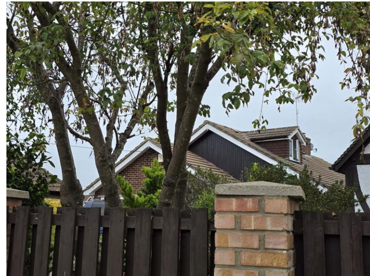
Existing roof dormer to be retained
