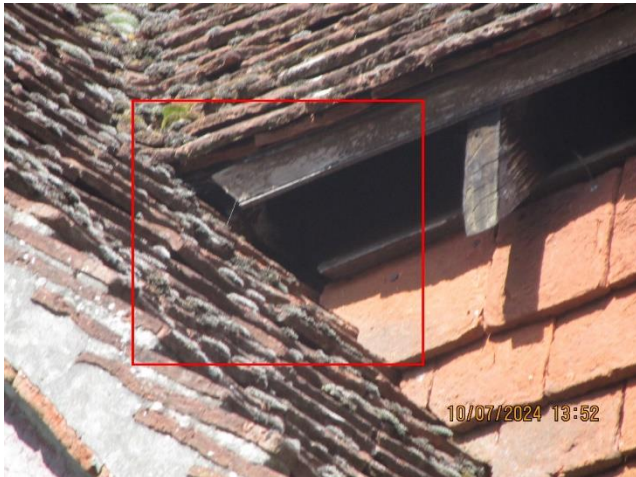
Photos 9 and 10 – Gaps under roof tiles
