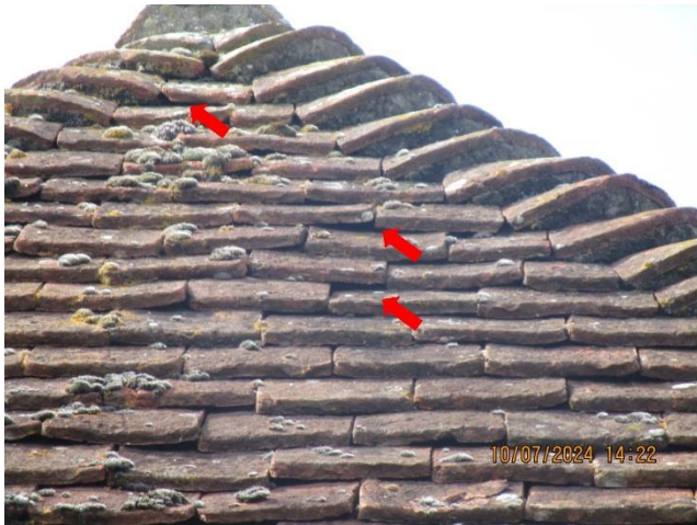
Photo 15 – Small gaps under the roof tiles of the garage, and Photo 16 – Inside the garage
