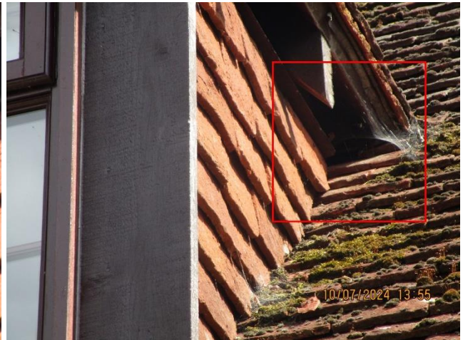
Photos 7 and 8– Gaps where the dormer windows join the main roof
