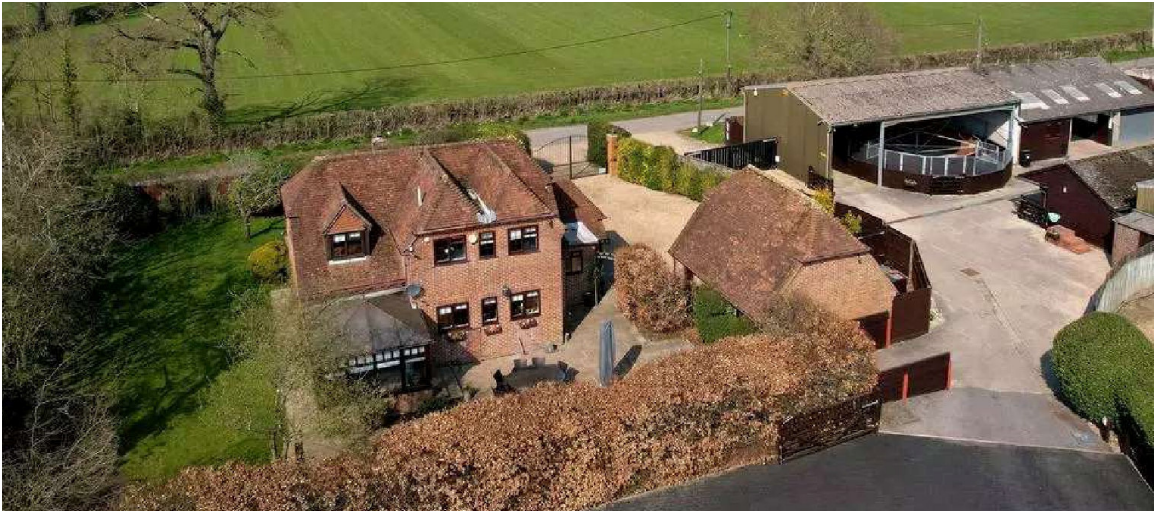
Fig 23078 05A View of rear elevation showing conservatory to be removed.
