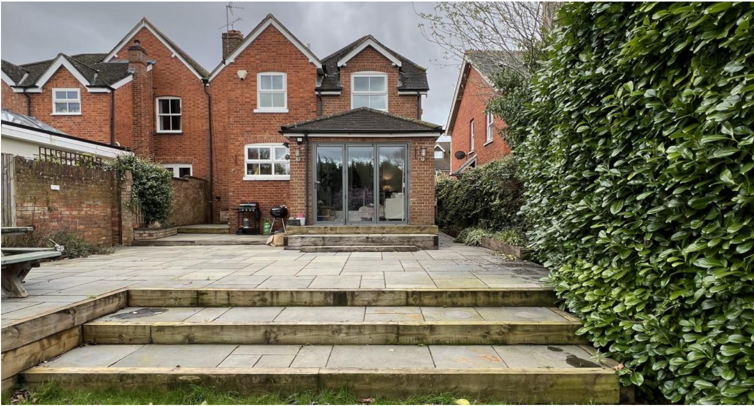
Photograph of existing rear
