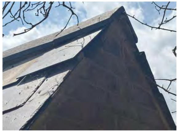
Plate 8 - PRFs on B2 in the form of a significant section of missing mortar at the verge edge.
