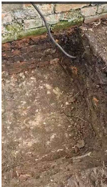
Photo 4a: Main House Foundation Trial Pit
