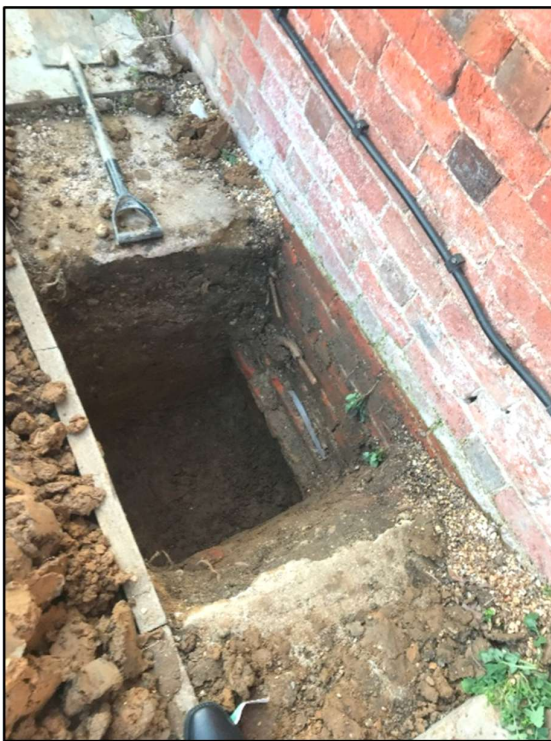
Photo 10 – Existing Cottage Foundation Check – Trial hole carried out near existing stairs.
