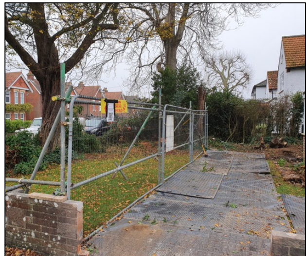
GP2: Tree protection barriers & trackmat ground protection
