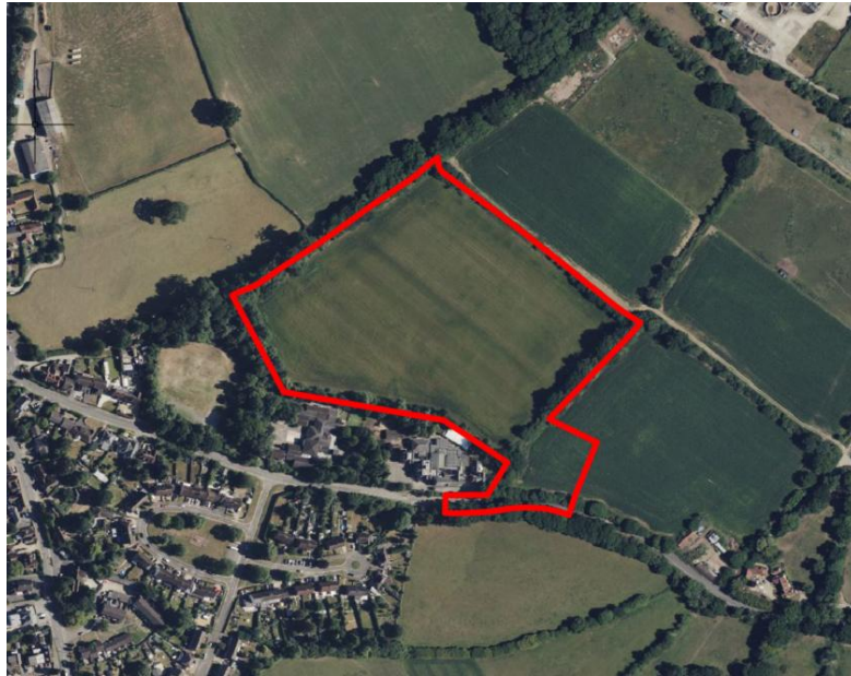
Figure 1: Site location shown on Google aerial image
