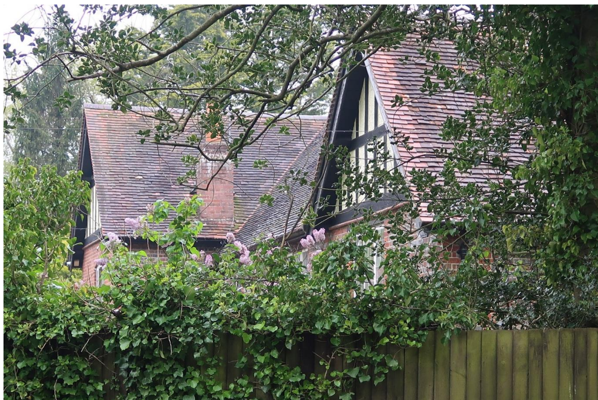
Figure 21 View of the roof and upper gables of Lanleypond Farmhouse from the south
