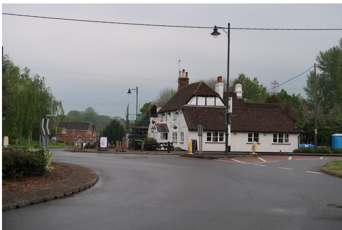
Figure 17 The Bull Public House adjacent the modern roundabout
