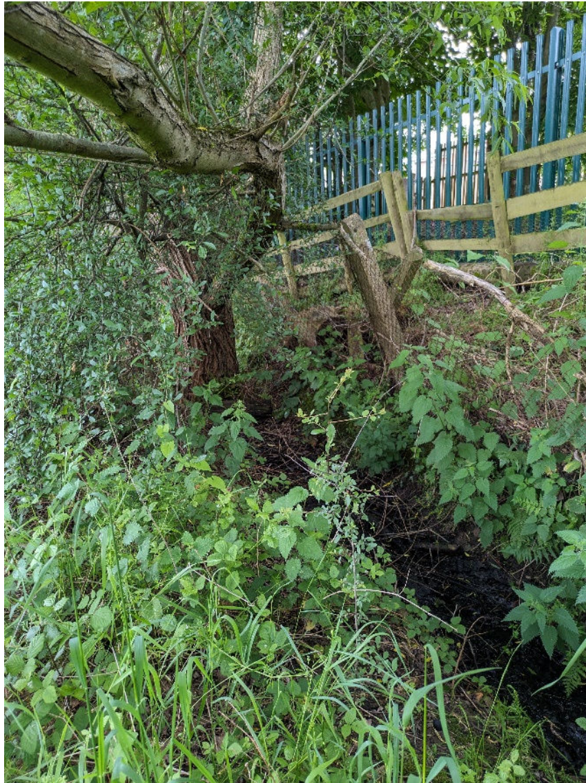
Figure 4: Southern watercourse adjacent to school boundary
