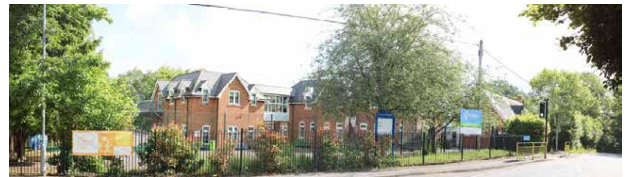
^Photo C - View from School Road adjacent to The Coombes Primary School
