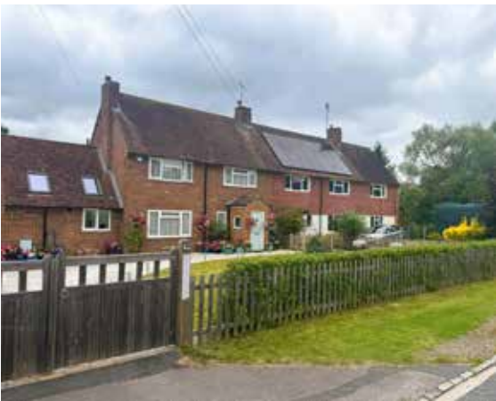
^Wide frontage semi-detached units with large courtyard parking
