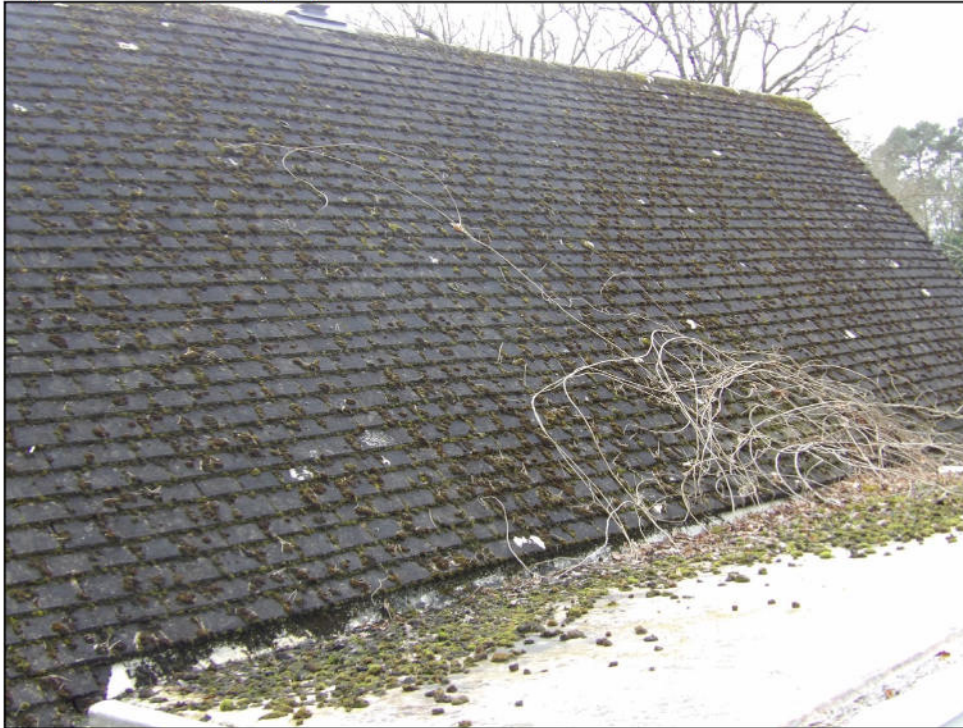
Figure 4. Example tightly fitted roof tiles. 5 Greenside, Crowthorne. 17.03.26
