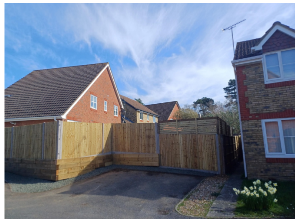
Figure 2 Site visit photo March 2026
