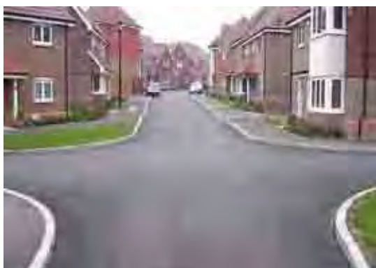
Figure 9.5 Four-way junction with no marked priority.
