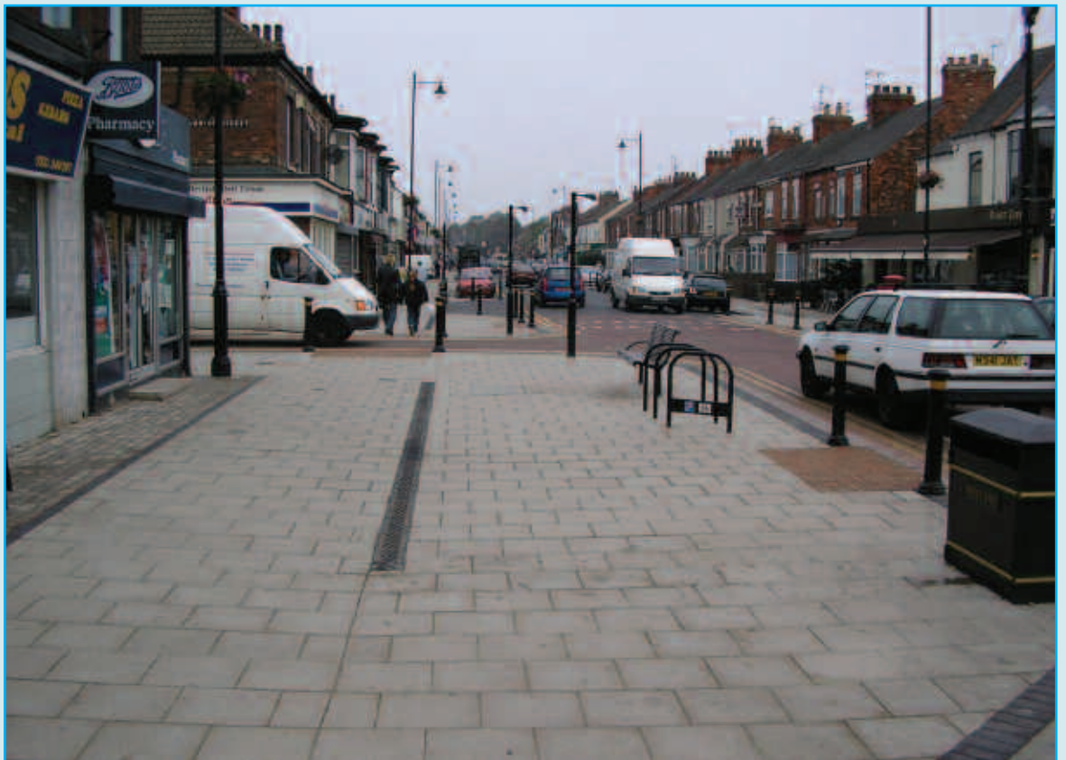
Footways widened significantly by narrowing carriageway
