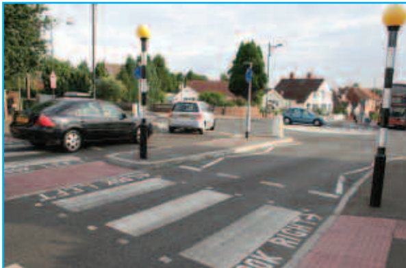
Zebra crossing close to mini-roundabout exit.
